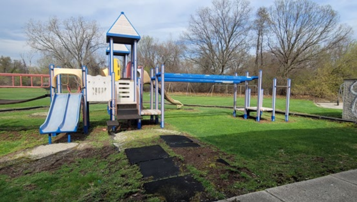
Playground - Before construction
