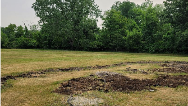
Playground - During construction
