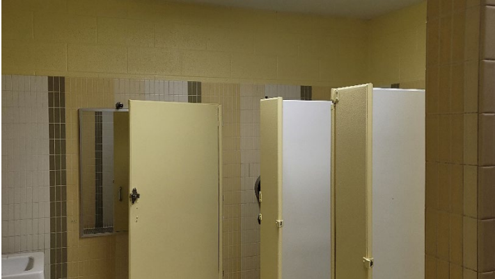
Toilet Room - During construction
