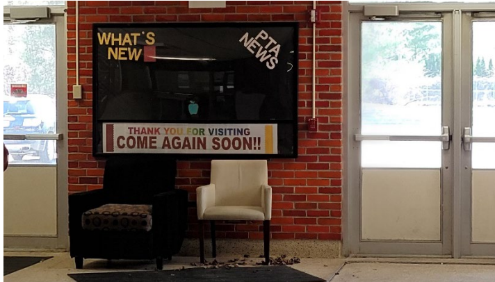
Lobby / Main Office - Before construction
