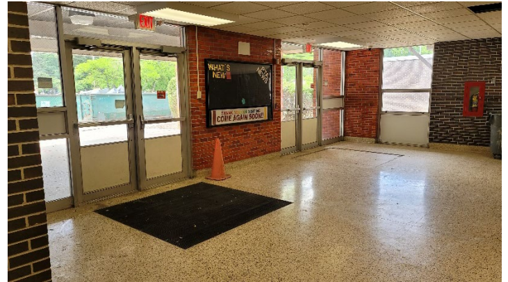
Lobby / Main Office - During construction
