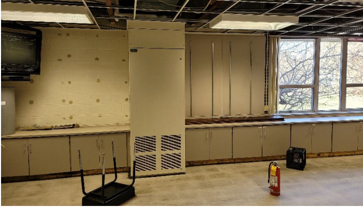
Classrooms - Before construction
