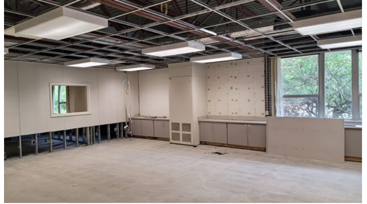
Classrooms - During construction
