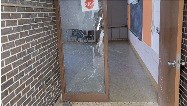
Common Areas - Before construction
