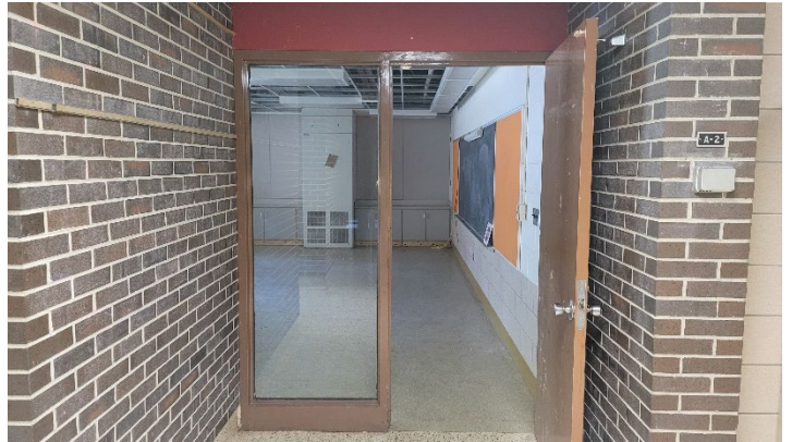
Common Areas - After construction
