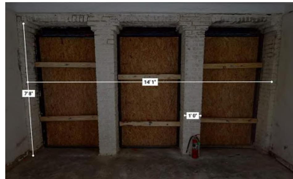
REF. PHOTO 1 - ARCADE ENTRANCE INTERIOR ELEVATION WEST
