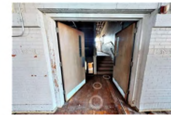
10B. NON-ACCESSIBLE CLASSROOM LEVEL (2ND FLOOR - SOUTH WING)
