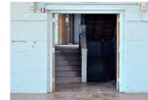
10A. NON-ACCESSIBLE CLASSROOM LEVEL (2ND FLOOR - NORTH WING)
