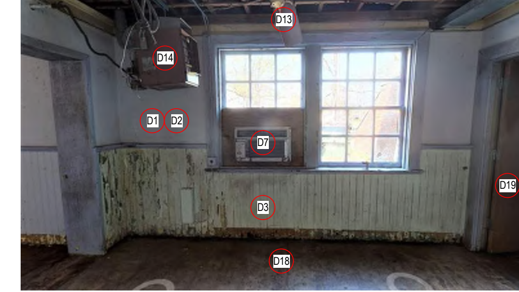
16 OFFICE 112A - WEST
