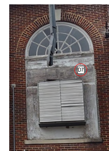
12 PLYWOOD INFILL & MECHANICAL LOUVER
