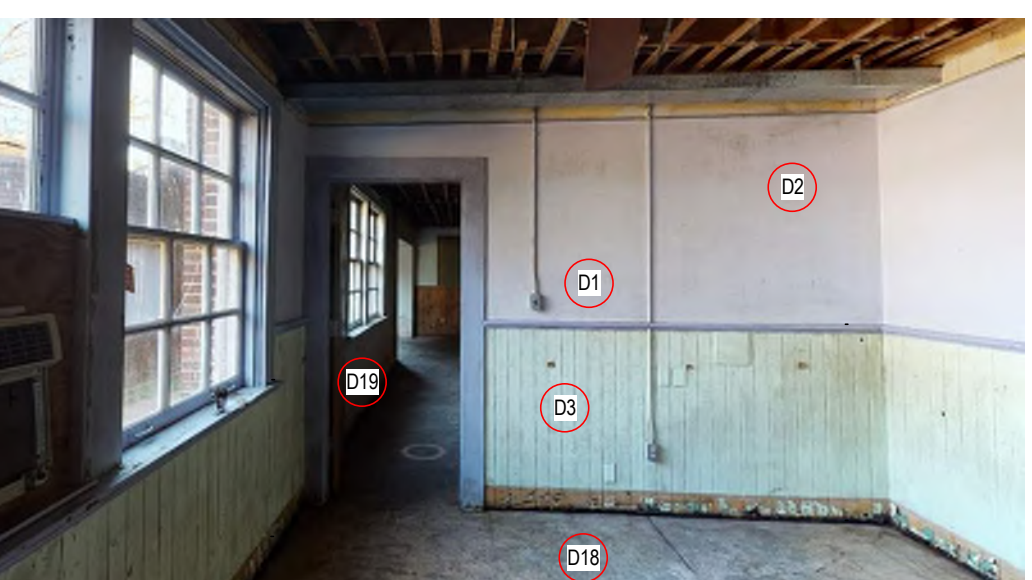
13 OFFICE 112A - NORTH
