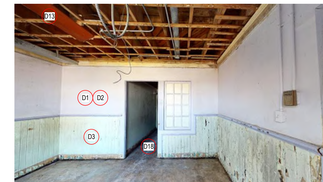
15 OFFICE 112A - EAST
