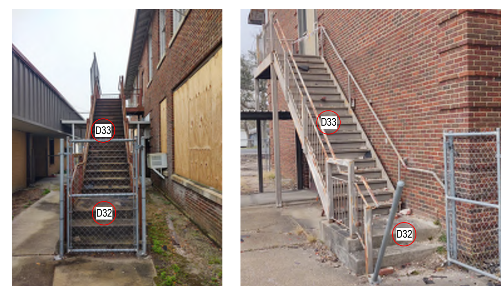
14 EXTERIOR METAL STAIRS NORTH EXTERIOR STAIR SOUTH EXTERIOR STAIR
