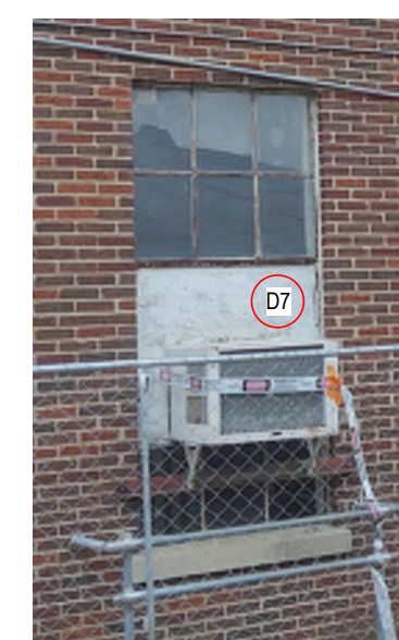
11 STEEL WINDOW & AC UNIT
