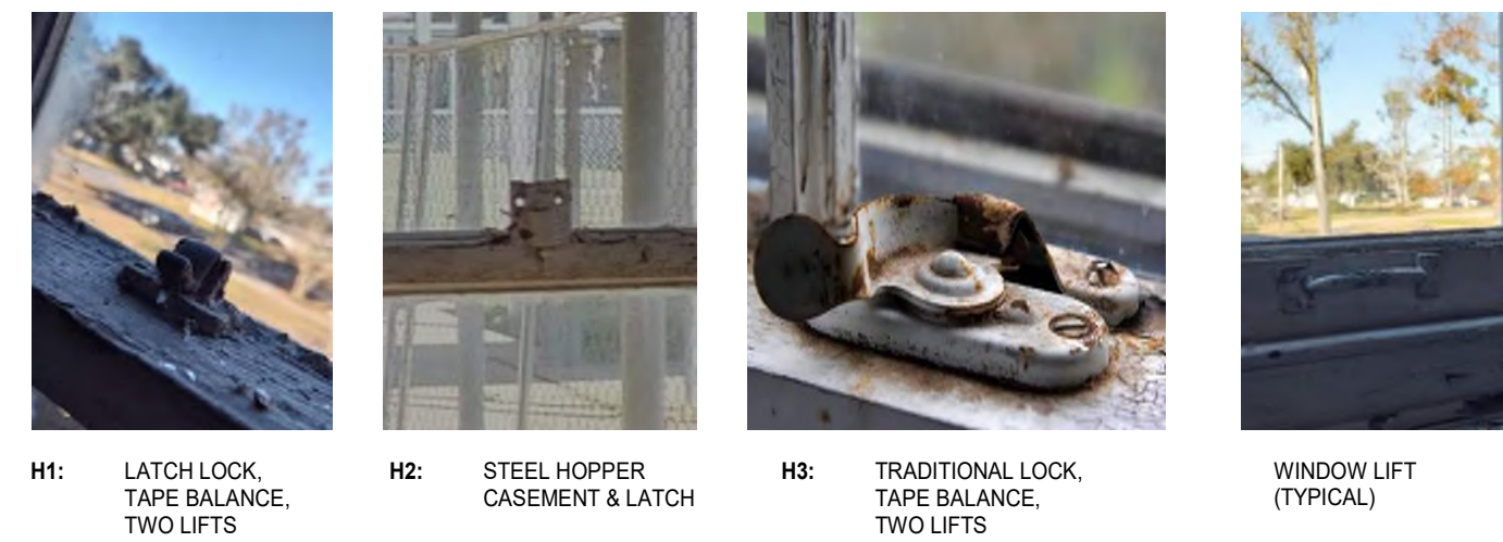
H1: LATCH LOCK, TAPE BALANCE, TWO LIFTS H2: STEEL HOPPER CASEMENT & LATCH H3: TRADITIONAL LOCK, TAPE BALANCE, TWO LIFTS WINDOW LIFT (TYPICAL)
