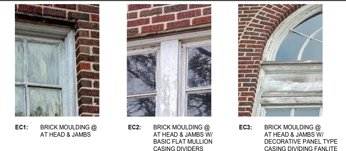
EC1: BRICK MOUNDING @ AT HEAD & JAMBS EC2: BRICK MOUNDING @ AT HEAD & JAMBS W/ BASIC FLAT MULLION CASING DIVIDERS EC3: BRICK MOUNDING @ AT HEAD & JAMBS W/ DECORATIVE PANEL TYPE CASING DIVIDING PANEL, FROM WINDOWS BENEATH
