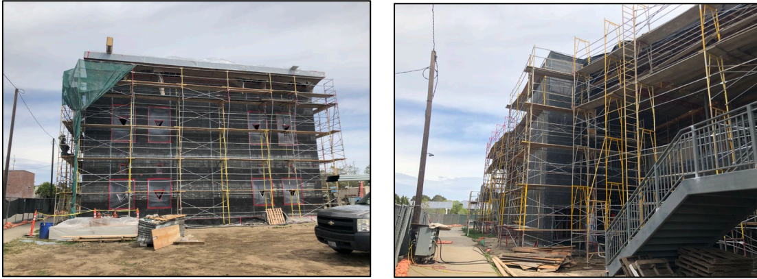
Marshall New Classroom Building Construction Progress – April 2019
