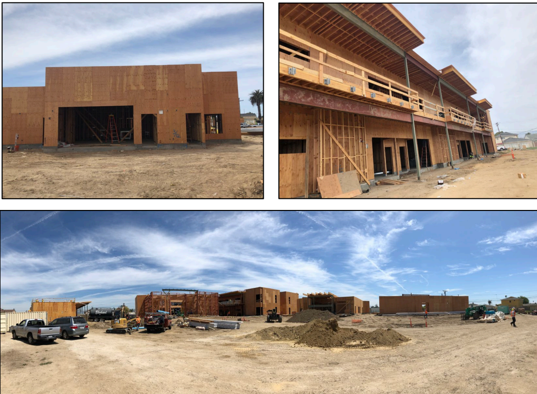
McKinna School Construction Progress – April 2019
