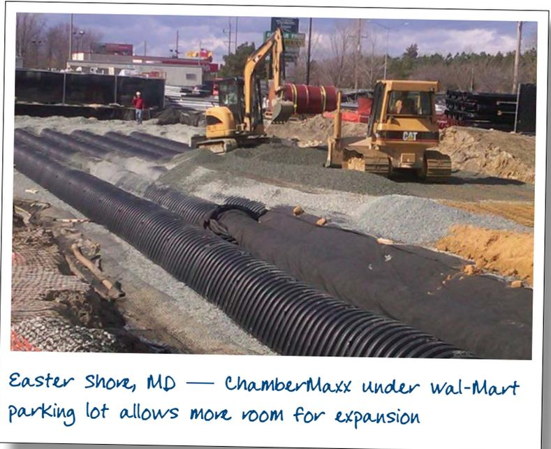
**The open-bottom chamber system allows for runoff reduction and economic infiltration**
