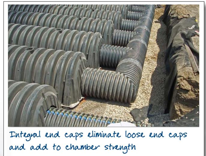
Integral end caps eliminate loose end caps and add to chamber strength
