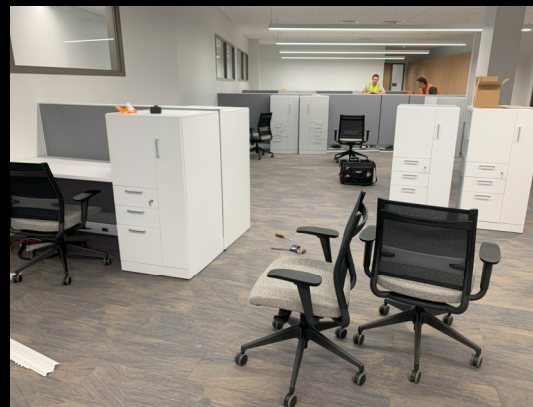
Furniture Installation Ongoing
