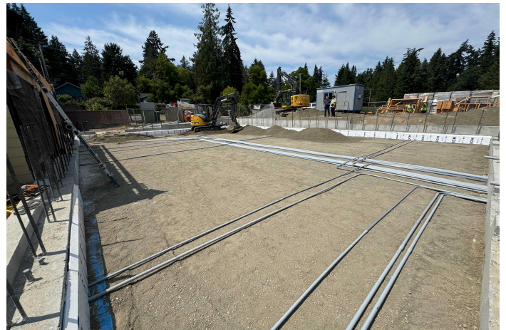
Underground electrical rough-in
