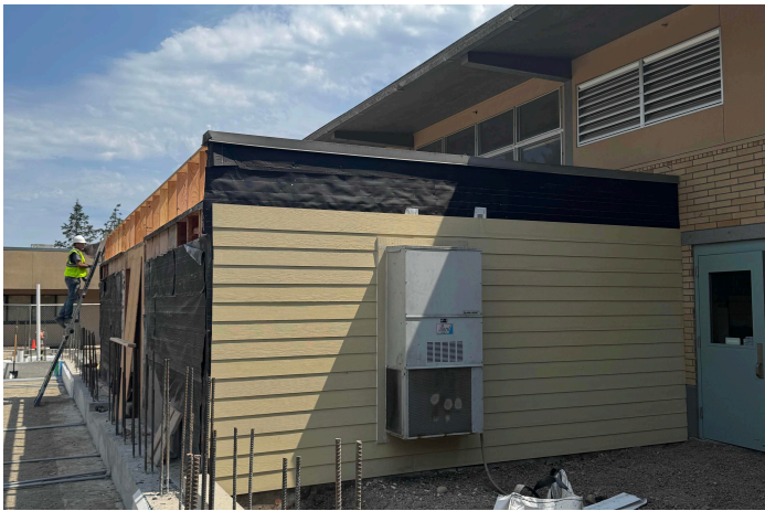
New siding installed
