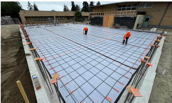
Vapor barrier and rebar installation
