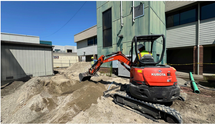
Sanitary sewer installation
