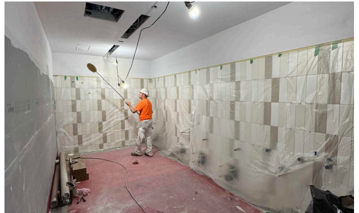
Tile installation and interior paint
