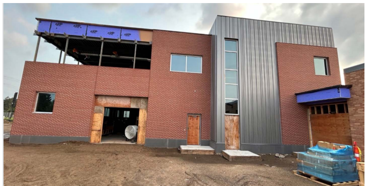
SLP Park Central Operations Center - Exterior
