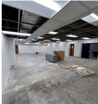
SLP High School Classroom Renovations Phase 2 - Classroom Progress
