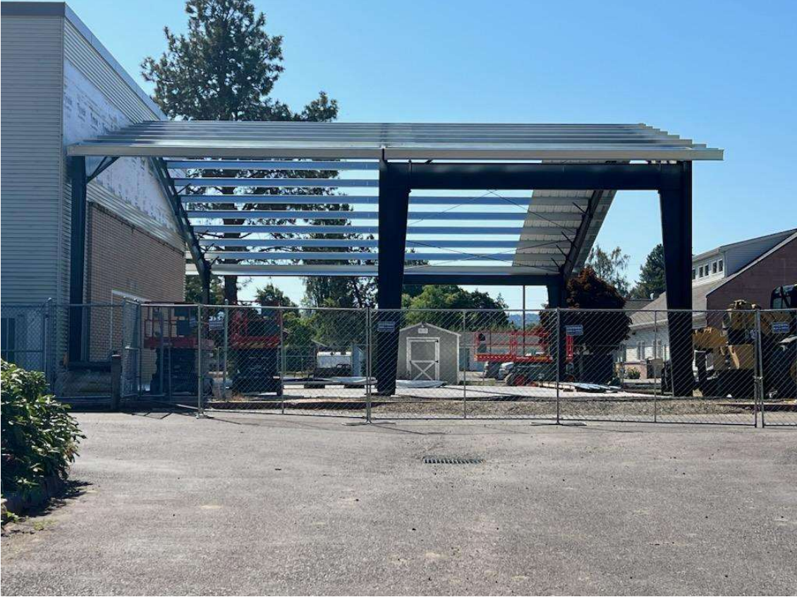
Clemens Primary School Play Shed:
