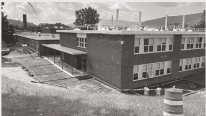
Newly improved sidewalks and drainage system at the Middle/High School.
