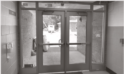
Woodstock Elementary School had a brand new exterior door installed.
