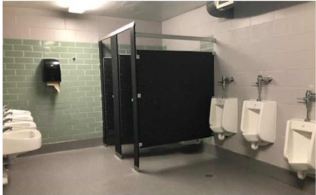
8.12.24 - Completed Boys Group Rest Room
