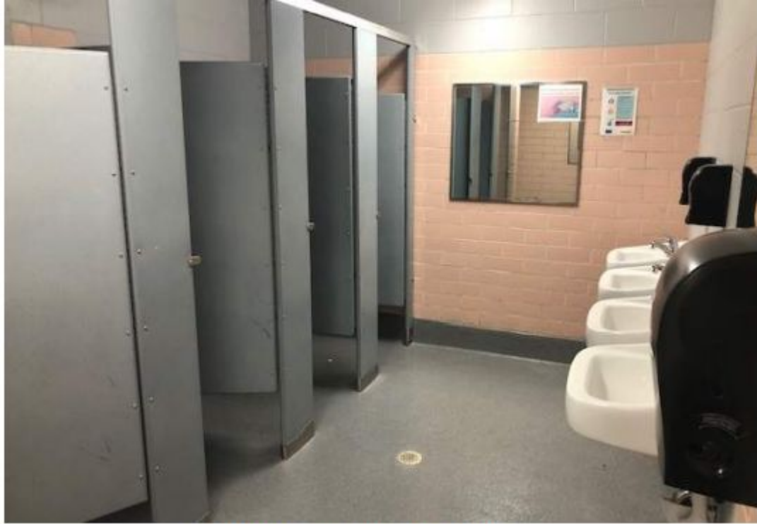
8.12.24 - Completed Girls Group Rest Room
