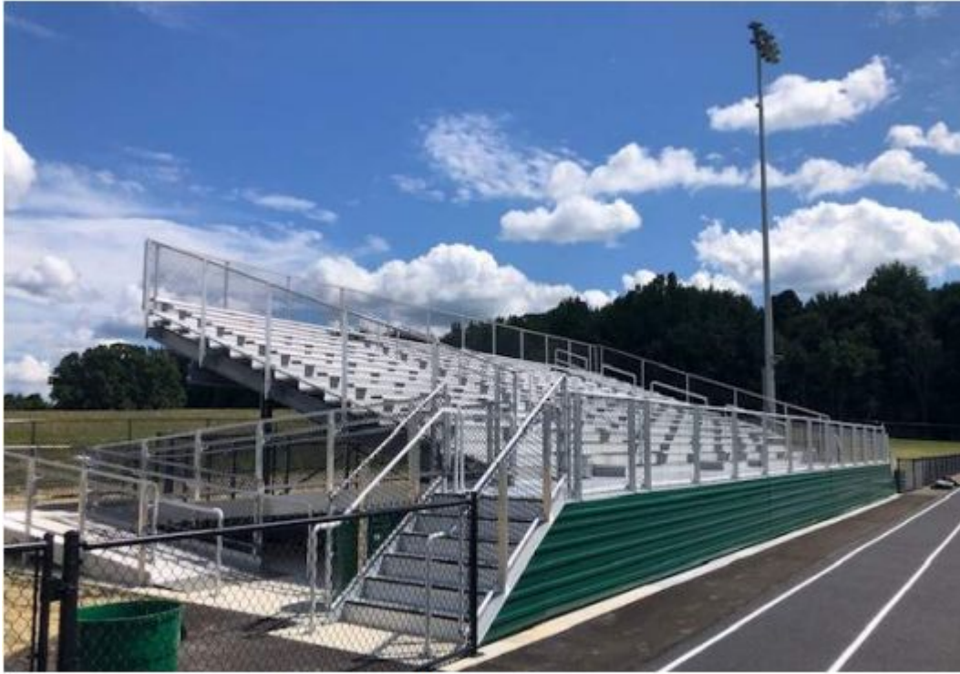
8.12.24 - Completed Visitor Grandstands
