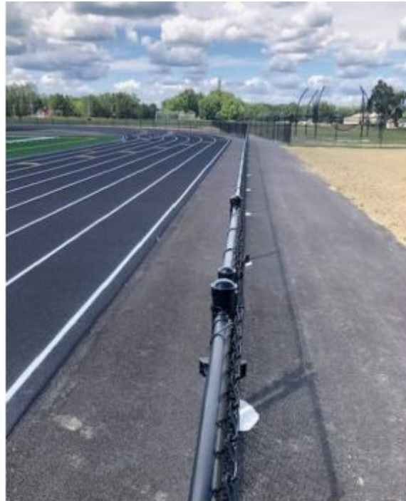
8.12.24 - Completed Fence, Final Seeding progress
