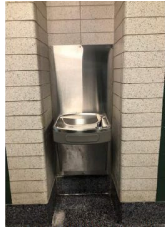
8.12.24 - Completed Drinking Fountain
