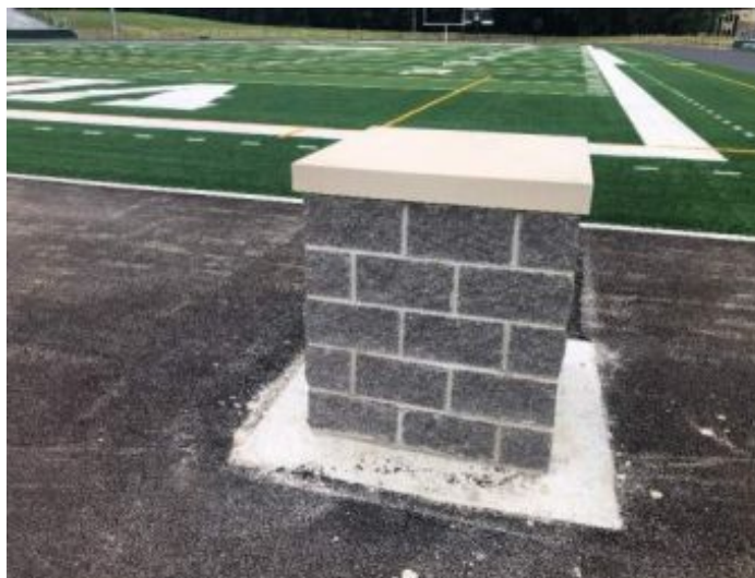
7.9.24 - Masonry Monument for Victory Bell
