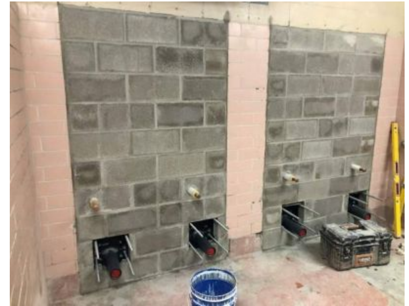
7.9.24 - Girl's Group Restroom, Masonry infil
