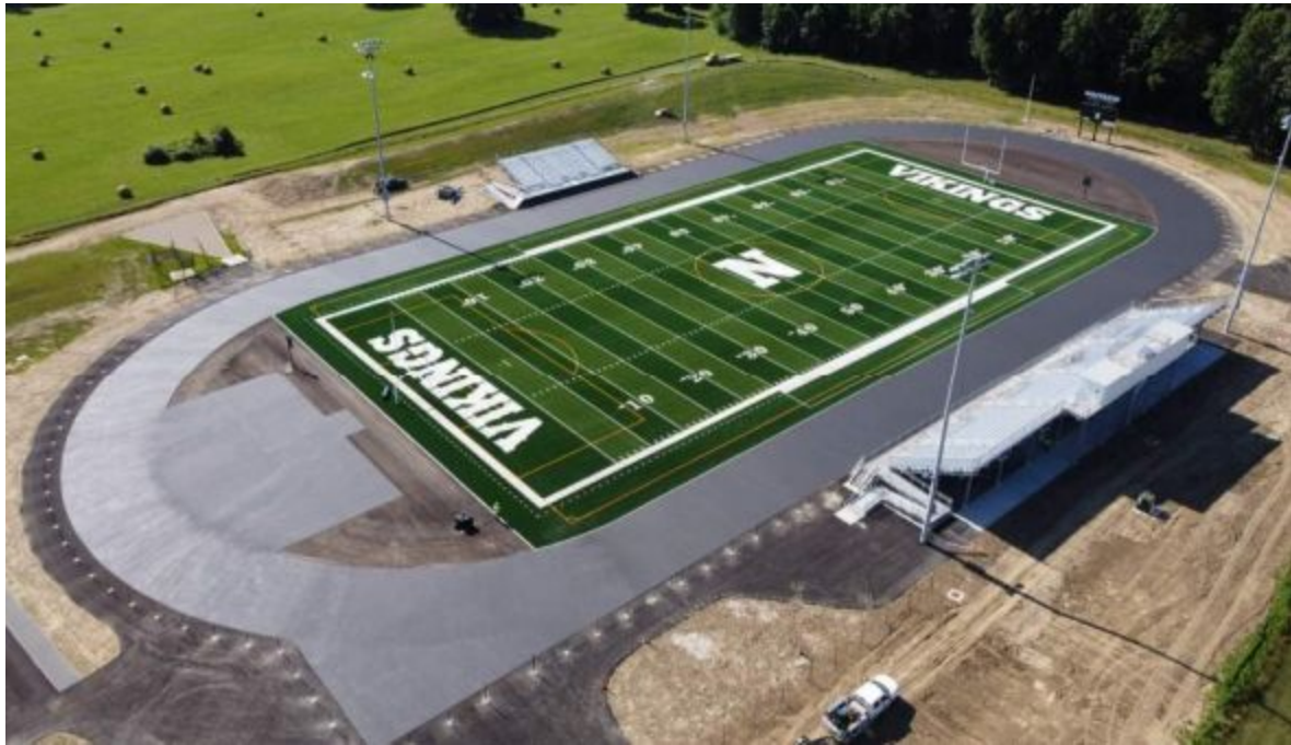
7.9.24 - Completed Track Surfacing, Turf Field, and Grandstands
