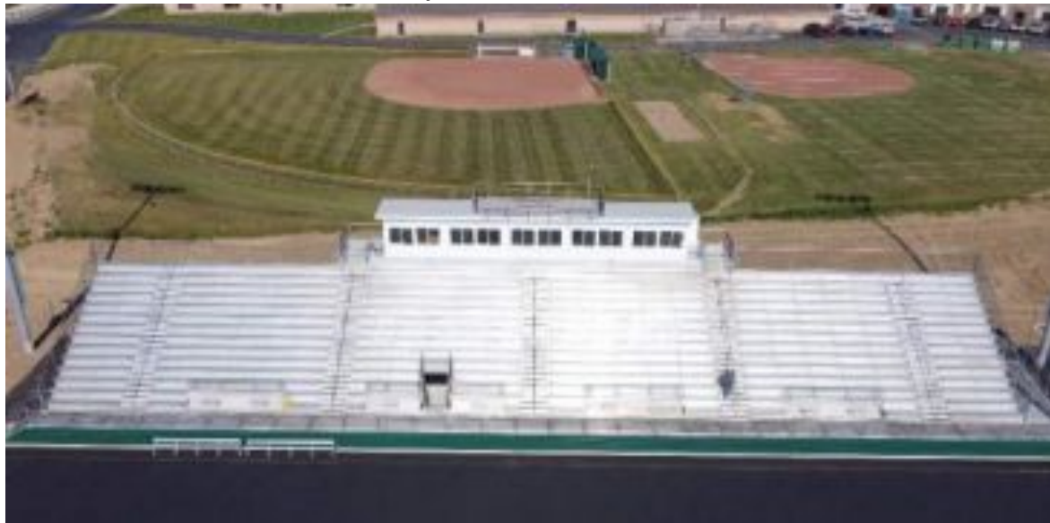
7.9.24 - Completed Home Grandstand
