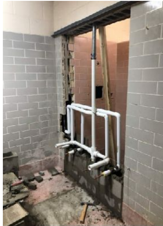
7.9.24 - Girls Locker Room, in wall plumbing and Masonry Infil
