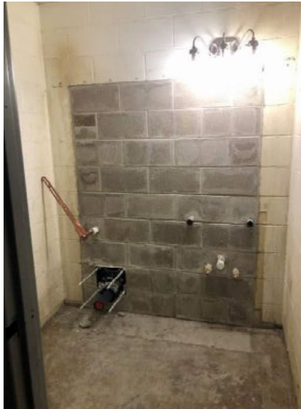
7.9.24 - Principal's Office Restroom, Masonry infil
