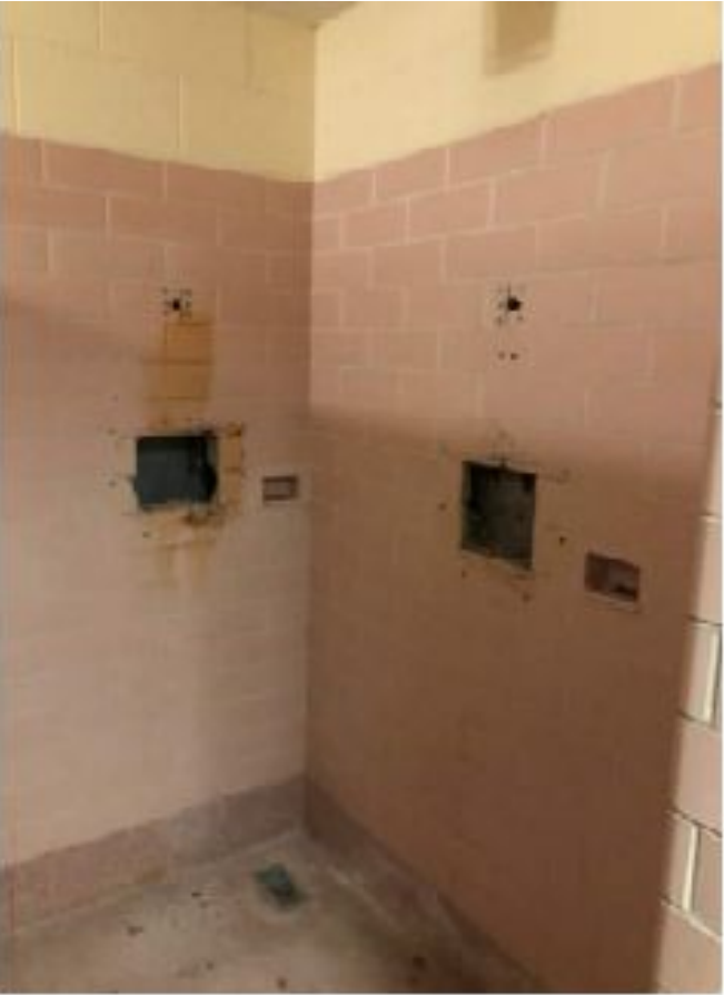
7.9.24 - Demolition of Fixtures at Boys Locker Room Shower
