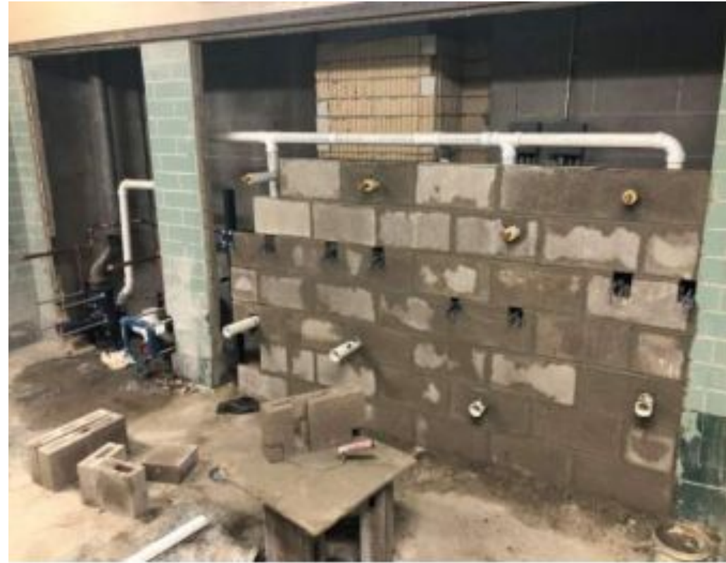
7.9.24 - In Wall Plumbing and Masonry Infil at Boys Group Restroom
