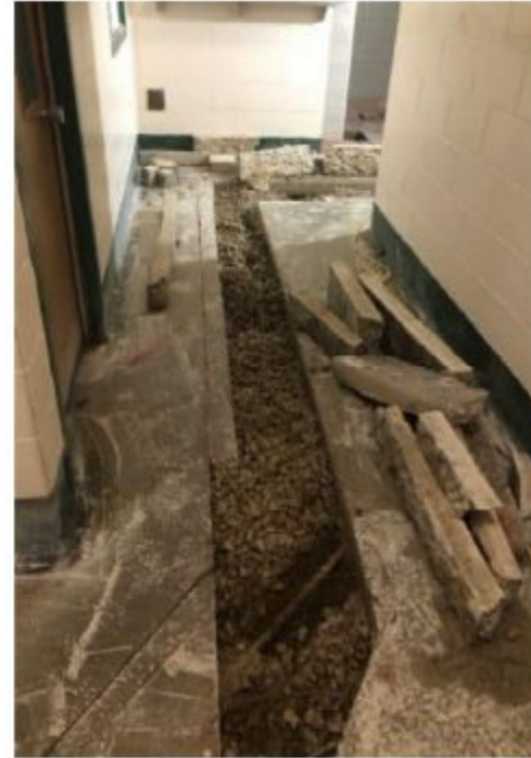
6.12.24 - MS Plumbing Repairs - Floor Demolition at Area 2 - Girls Locker Room
