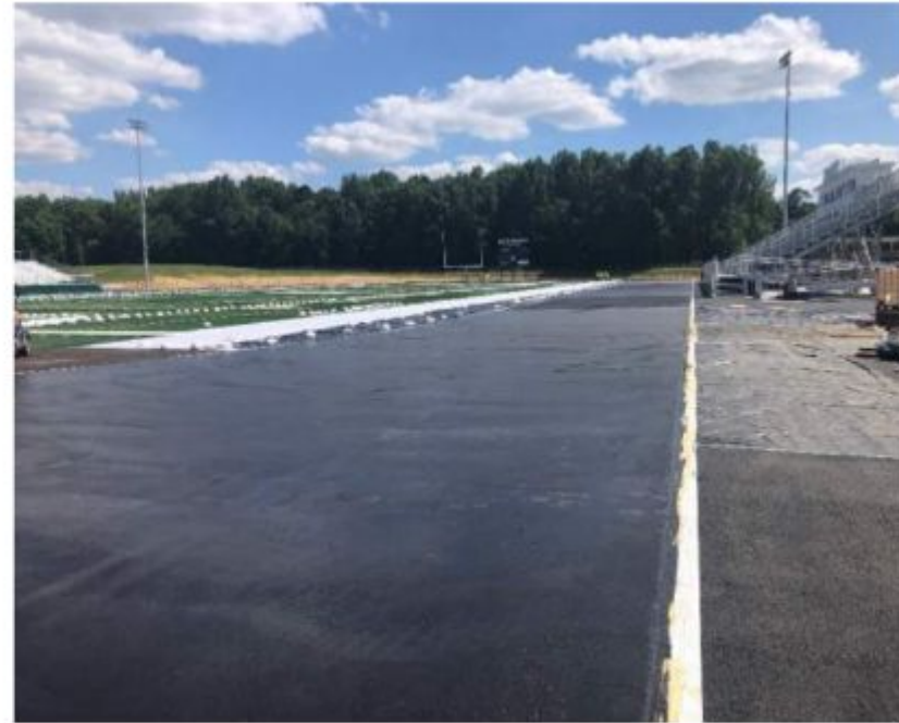
6.11.24 - Track Surfacing Progress
