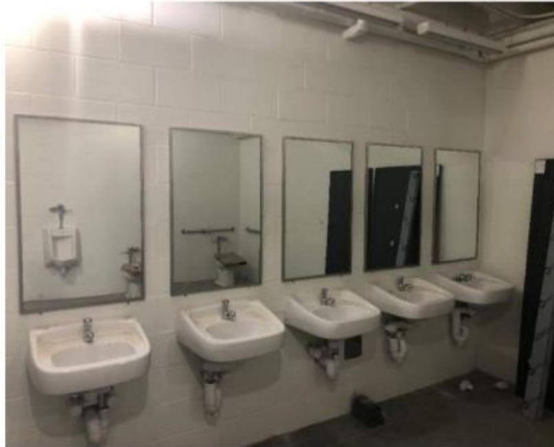
6.11.24 - Mirrors & Lavatory Sinks at Men's Restroom
