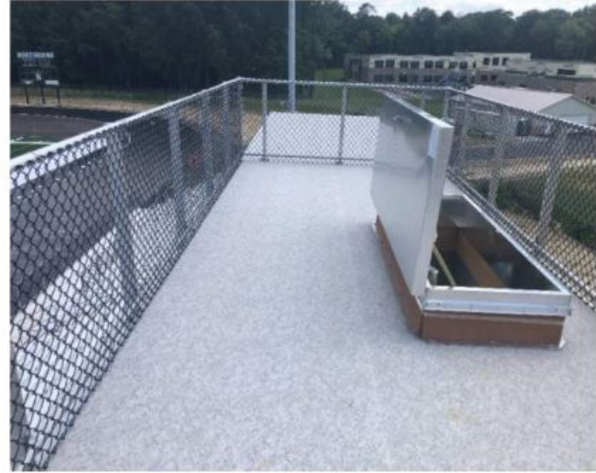
6.11.24 - Roof Top Camera Platform at Press Box
