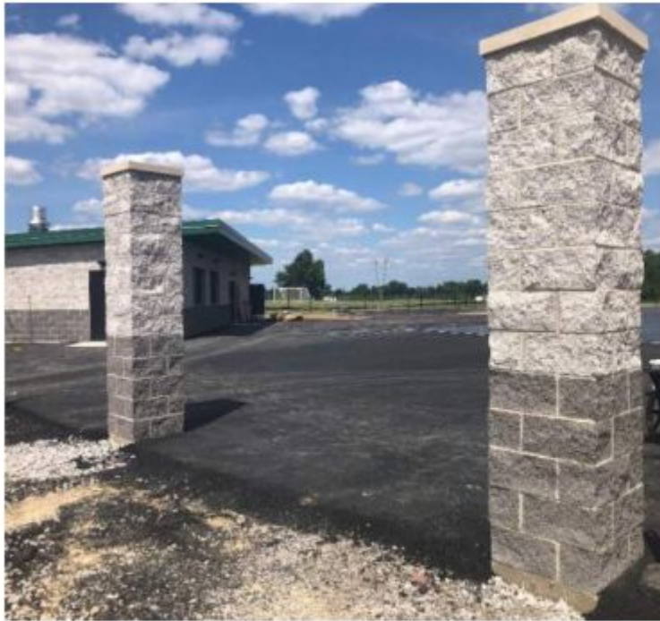
6.11.24 - Masonry Piers for Entry Gates
