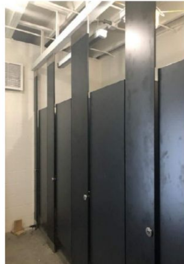
6.11.24 - Toilet Partitions at Women's Restroom
