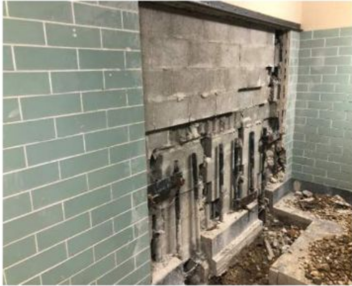
6.12.24 - Middle School Plumbing Repairs - Floor and Wall Demolition at Area 4 - Boys Group Restroom
