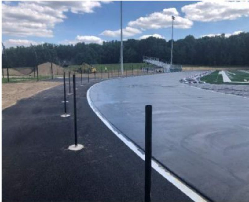
06.11.24 - Track Surfacing Progress & 4' Fence Posts
