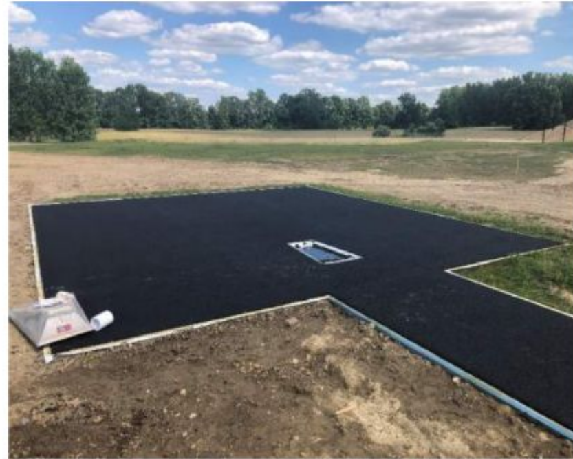
06.11.24 - Track Surfacing Base Course at Pole Vault
