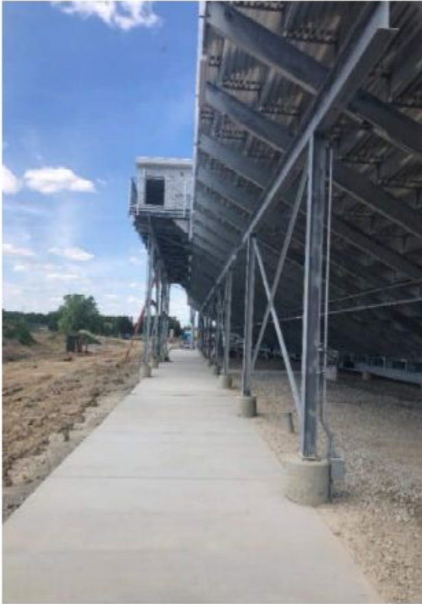
6.11.24 - Electrical Conduits, Lights, and Concrete Walk at Home Grandstands
