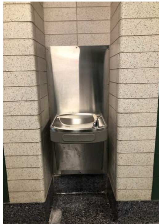
8.12.24 - Completed Drinking Fountain
