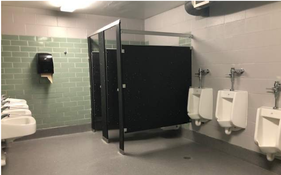
8.12.24 - Completed Boys Group Rest Room
