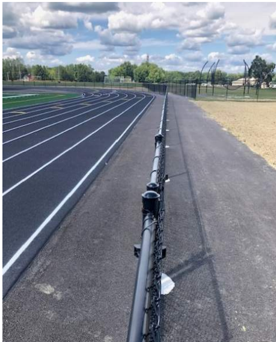
8.12.24 - Completed Fence, Final Seeding progress
