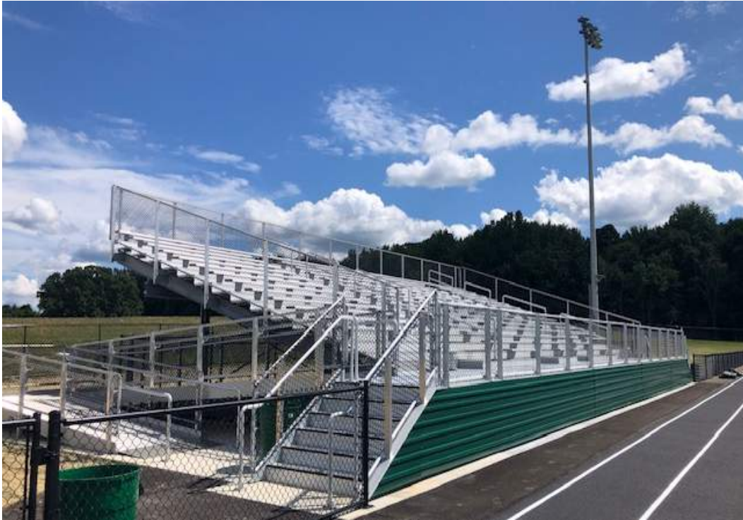
8.12.24 - Completed Visitor Grandstands
