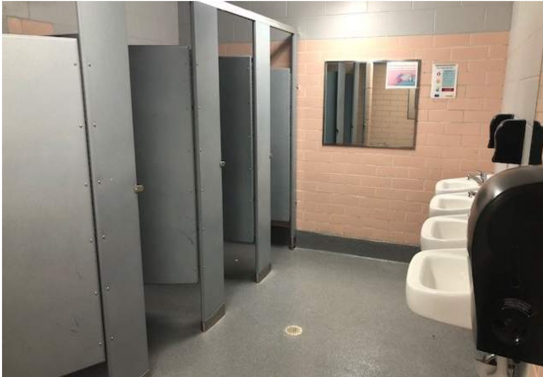
8.12.24 - Completed Girls Group Rest Room
