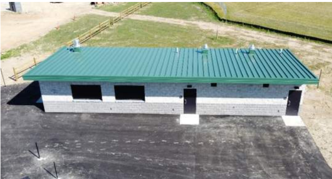
7.9.24 - Completed Concession Stand
