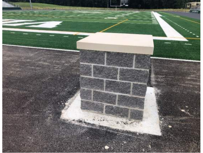
7.9.24 - Masonry Monument for Victory Bell
