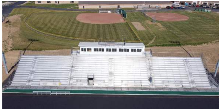
7.9.24 - Completed Home Grandstand
