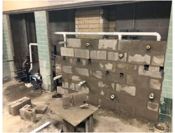
7.9.24 - In Wall Plumbing and Masonry Infil at Boys Group Restroom
