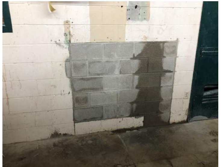
7.9.24 - Masonry Infil at Shop Classroom
