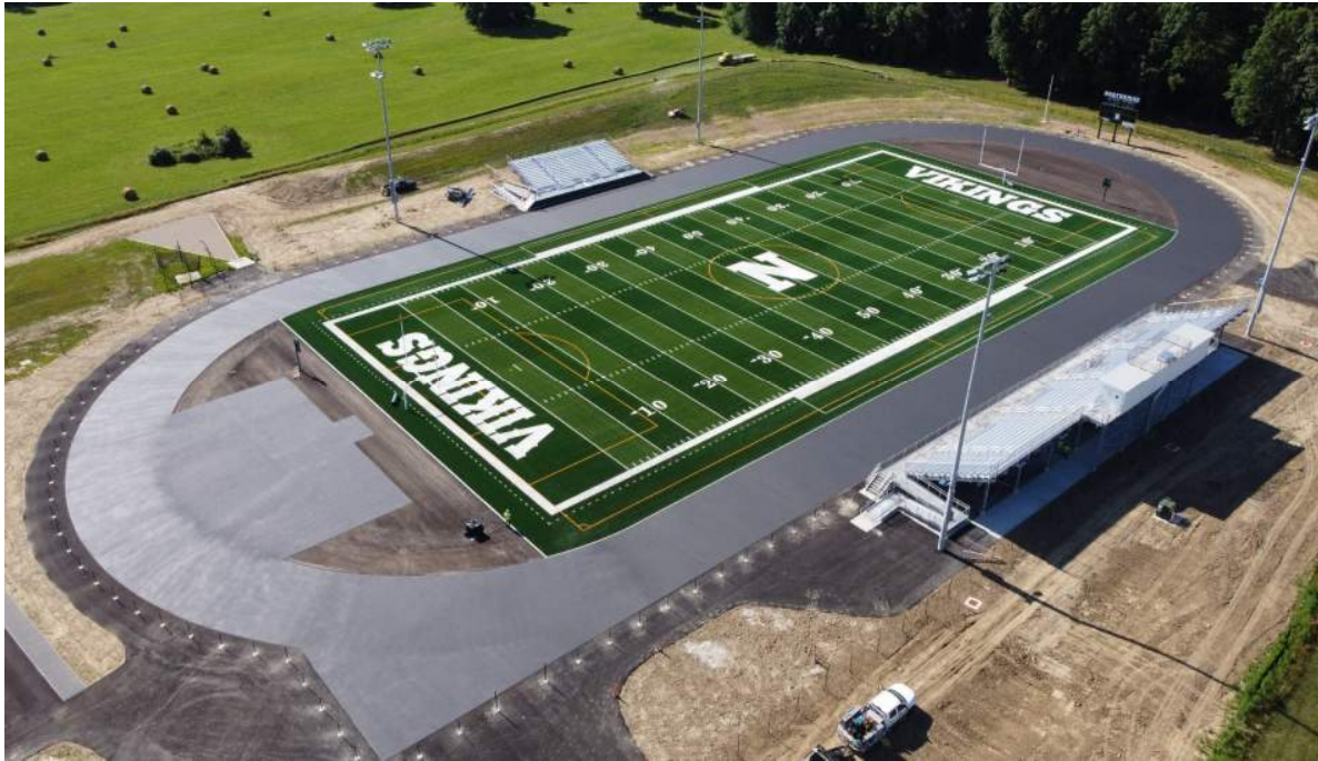
7.9.24 - Completed Track Surfacing, Turf Field, and Grandstands
