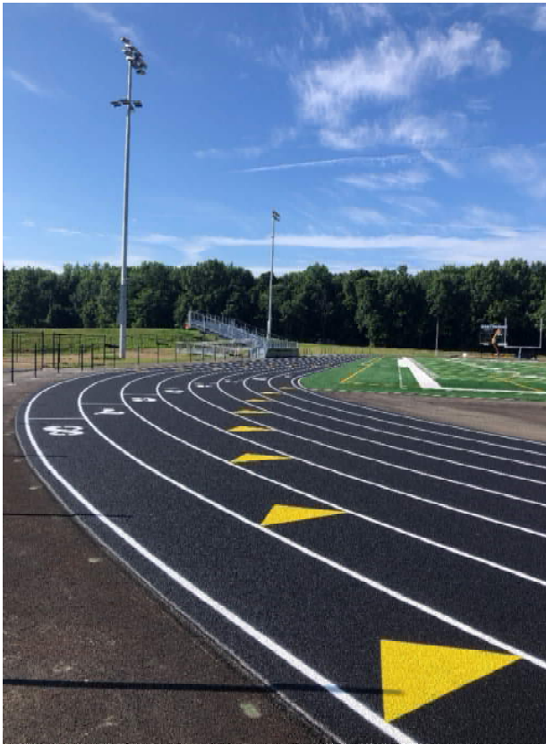
7.9.24 - Lane Markings at Track
