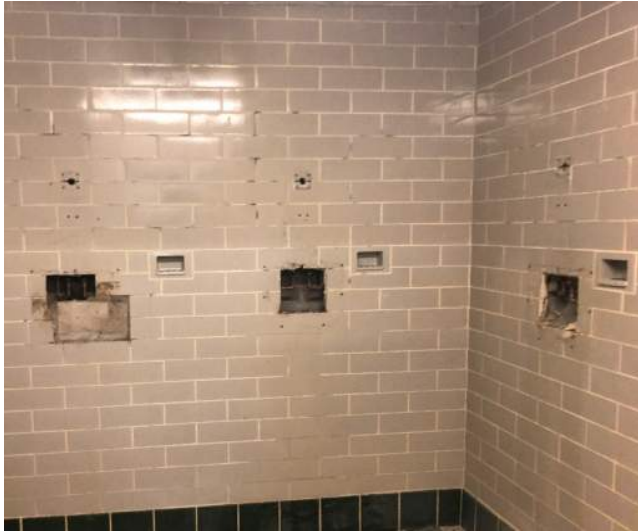
7.9.24 - Demolition of Fixtures at Boys Locker Room Shower
