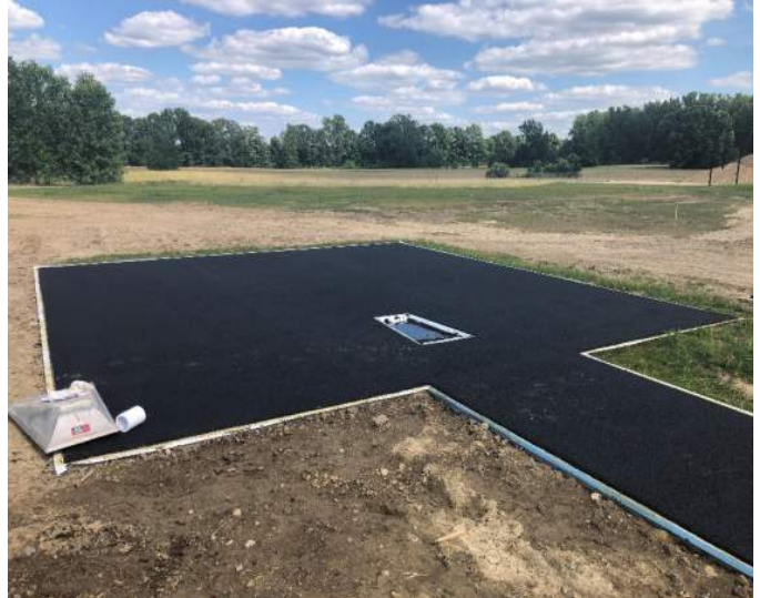
06.11.24 - Track Surfacing Base Course at Pole Vault
