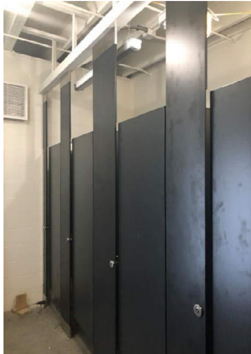
6.11.24 - Toilet Partitions at Women's Restroom
