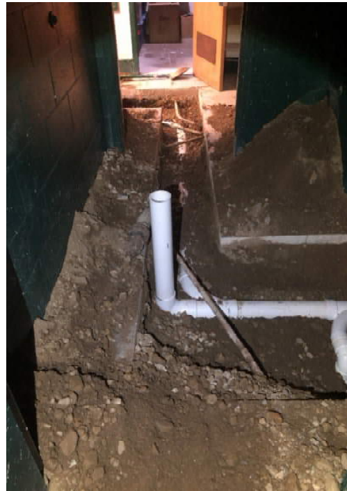
6.12.24 - MS Plumbing Repairs - New Underground Sanitary Line at Area 1 - Boys Locker Room
