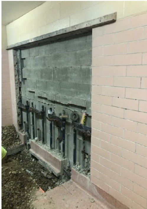
6.12.24 - MS Plumbing Repairs - Floor & Wall Demolition at Area 3 - Girls Group Restroom
