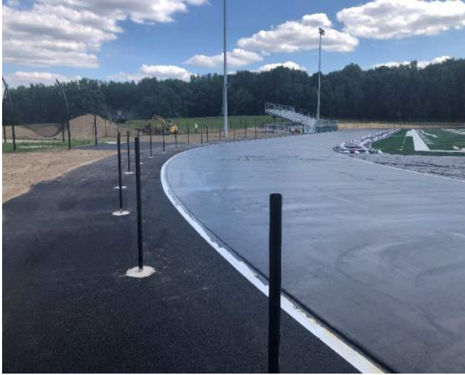
06.11.24 - Track Surfacing Progress & 4' Fence Posts
