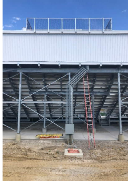
6.11.24 - Conduit for Data and Audio to Press Box
