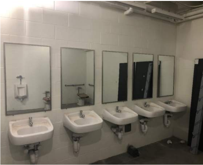
6.11.24 - Mirrors & Lavatory Sinks at Men's Restroom
