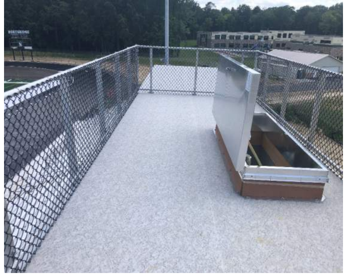
6.11.24 - Roof Top Camera Platform at Press Box
