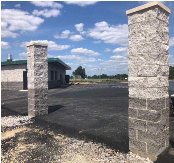
6.11.24 - Masonry Piers for Entry Gates
