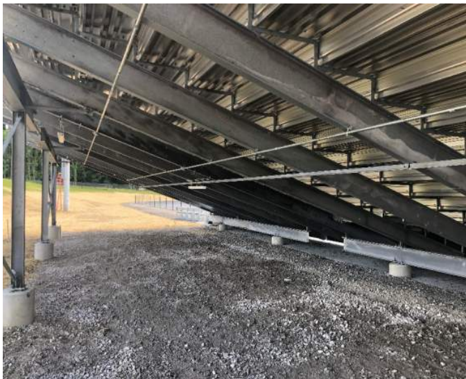
6.11.24 - Electrical Conduit and Lights at Visitor Grandstands
