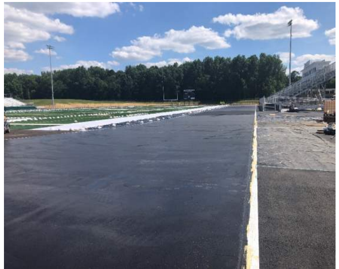
6.11.24 - Track Surfacing Progress
