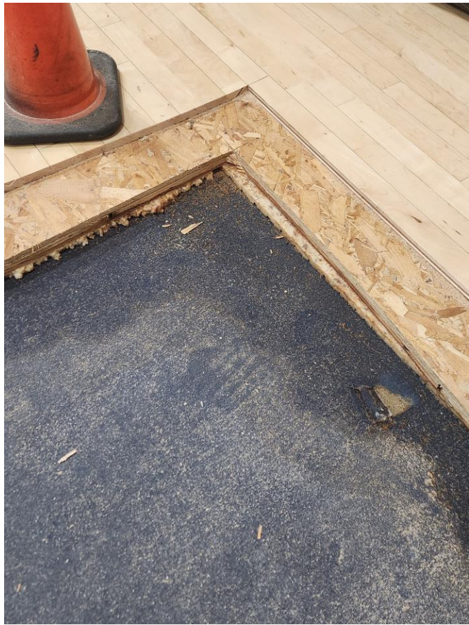
Gym floor repair of water damage from roof leak at AMSO
