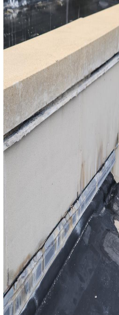
Coping Stone deterioration at ARHS
