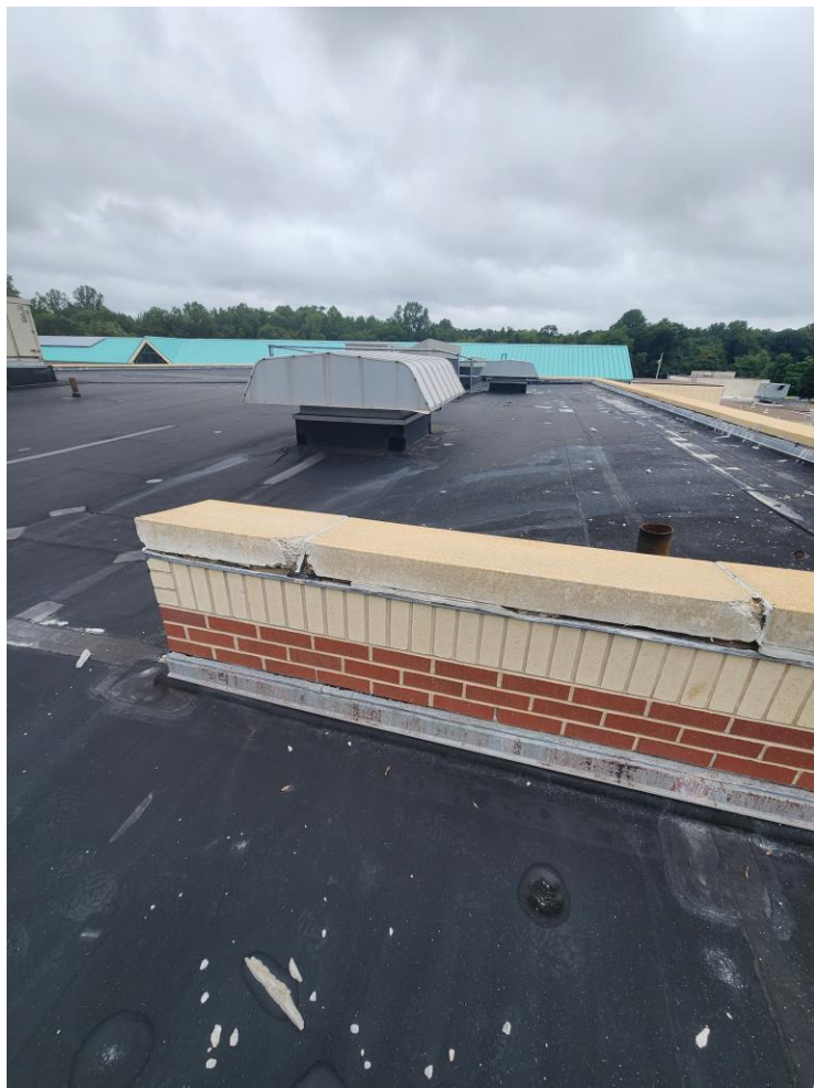
Coping Stone deterioration at ARHS
