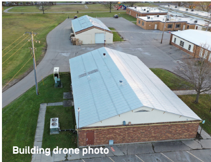
Building drone photo
