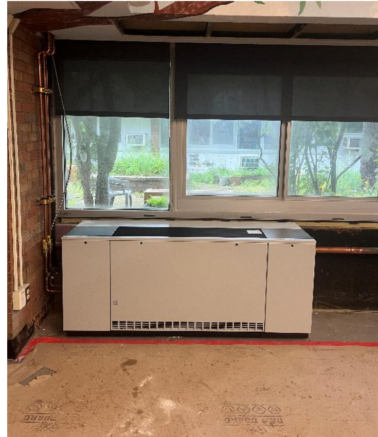
Library Mechanical Upgrades
