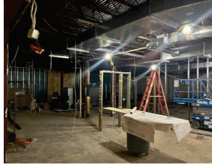
1964 (Area A) Progress
