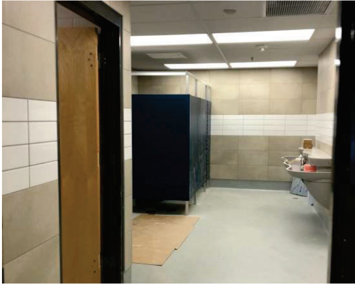
Restroom Build Back
