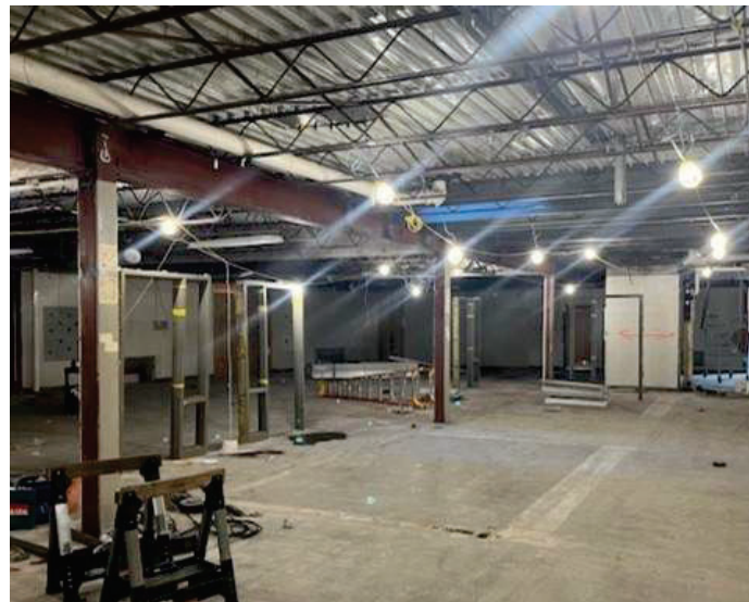
1964 (Area A) Progress
