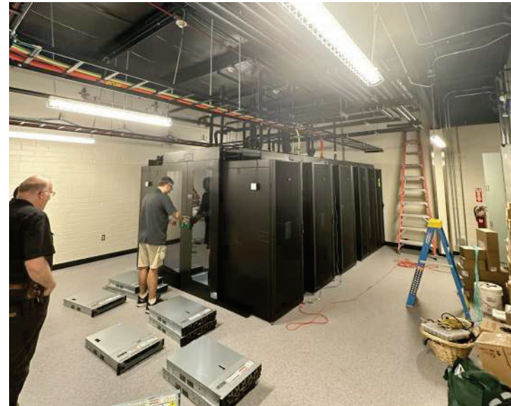
Data Pod Install
