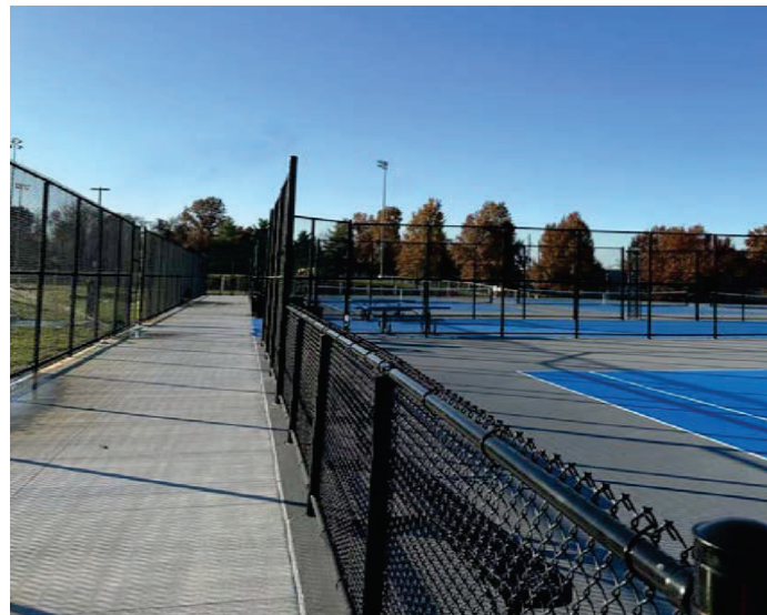
East Concourse Looking South
