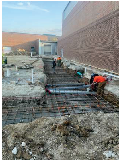
DMS - Footing Rebar
