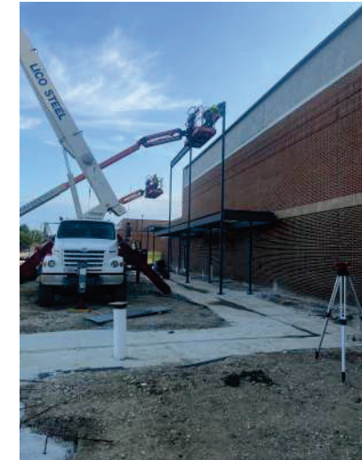
SVMS - Steel Erection
