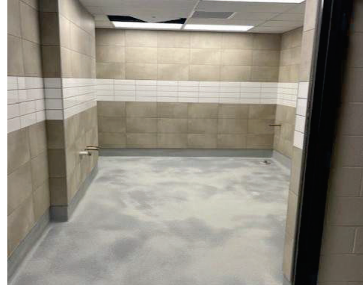
Restroom Build Back
