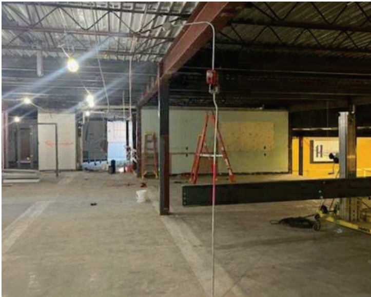
1964 (Area A) Progress
