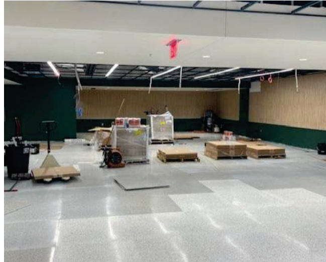
Cafeteria Build Back
