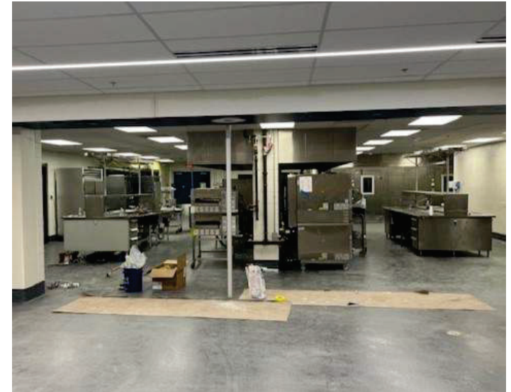
Kitchen Build Back
