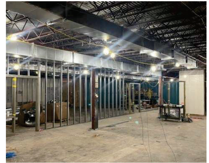
1964 (Area A) Progress
