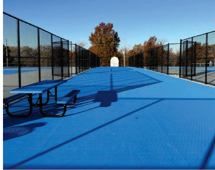
Center Spectator Concourse Looking West
