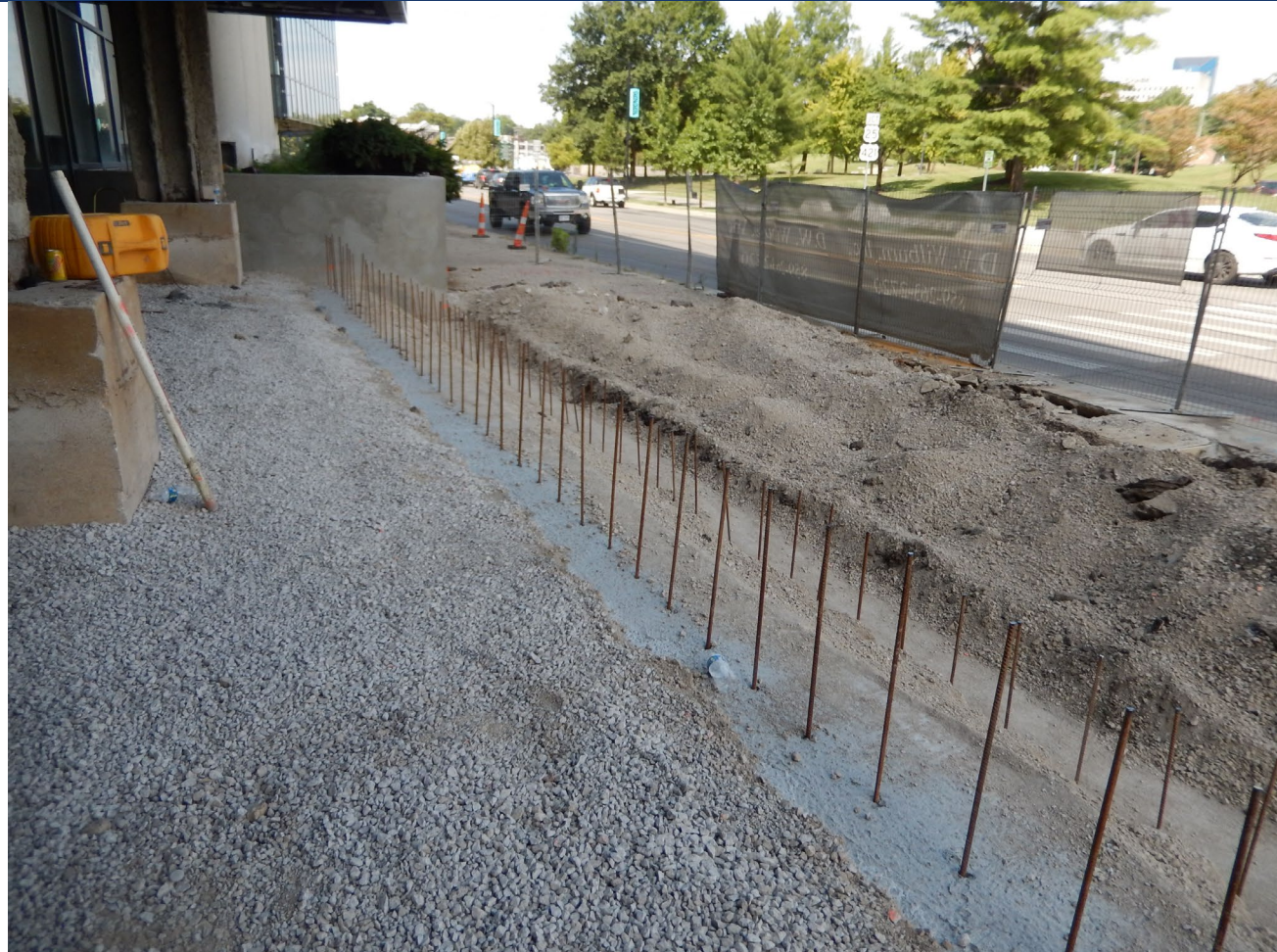
Midland entry stair foundations
