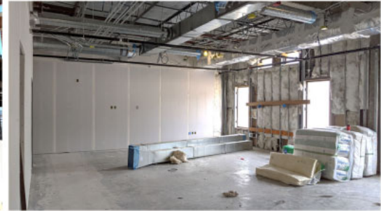
Classroom addition underway in renovated library
