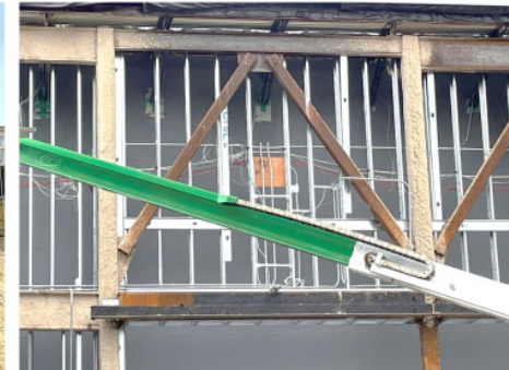
Partial demolition at cafeteria
