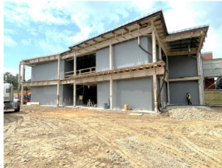
Demolition complete at classroom wing
