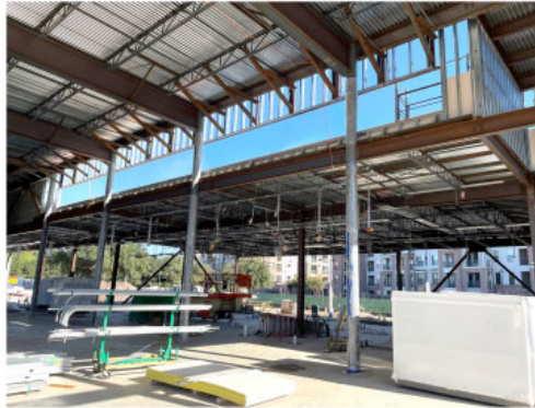
Clerestory opening at cafeteria
