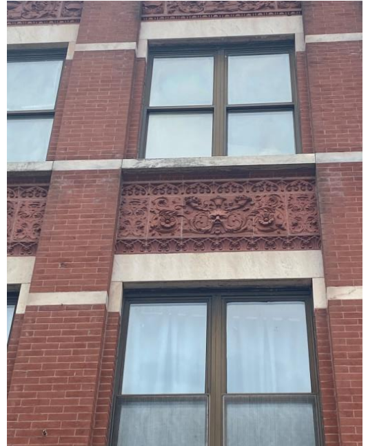
This terra cotta panel at 246 Main Street is a primary material as well as a decorative architectural feature.
