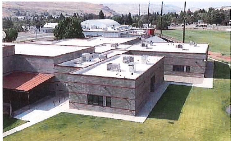
New addition to Okanogan High School includes two new classrooms.
