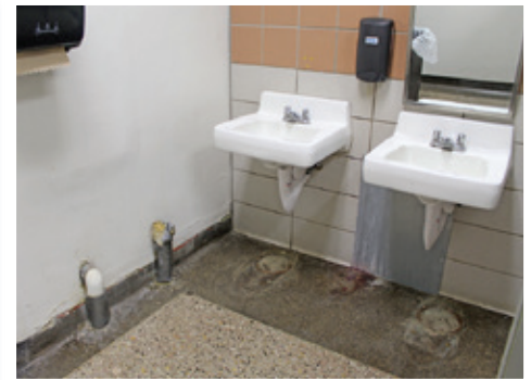
Existing second floor bathroom
