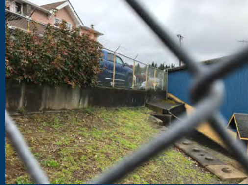
Stewart Field Retaining Wall
