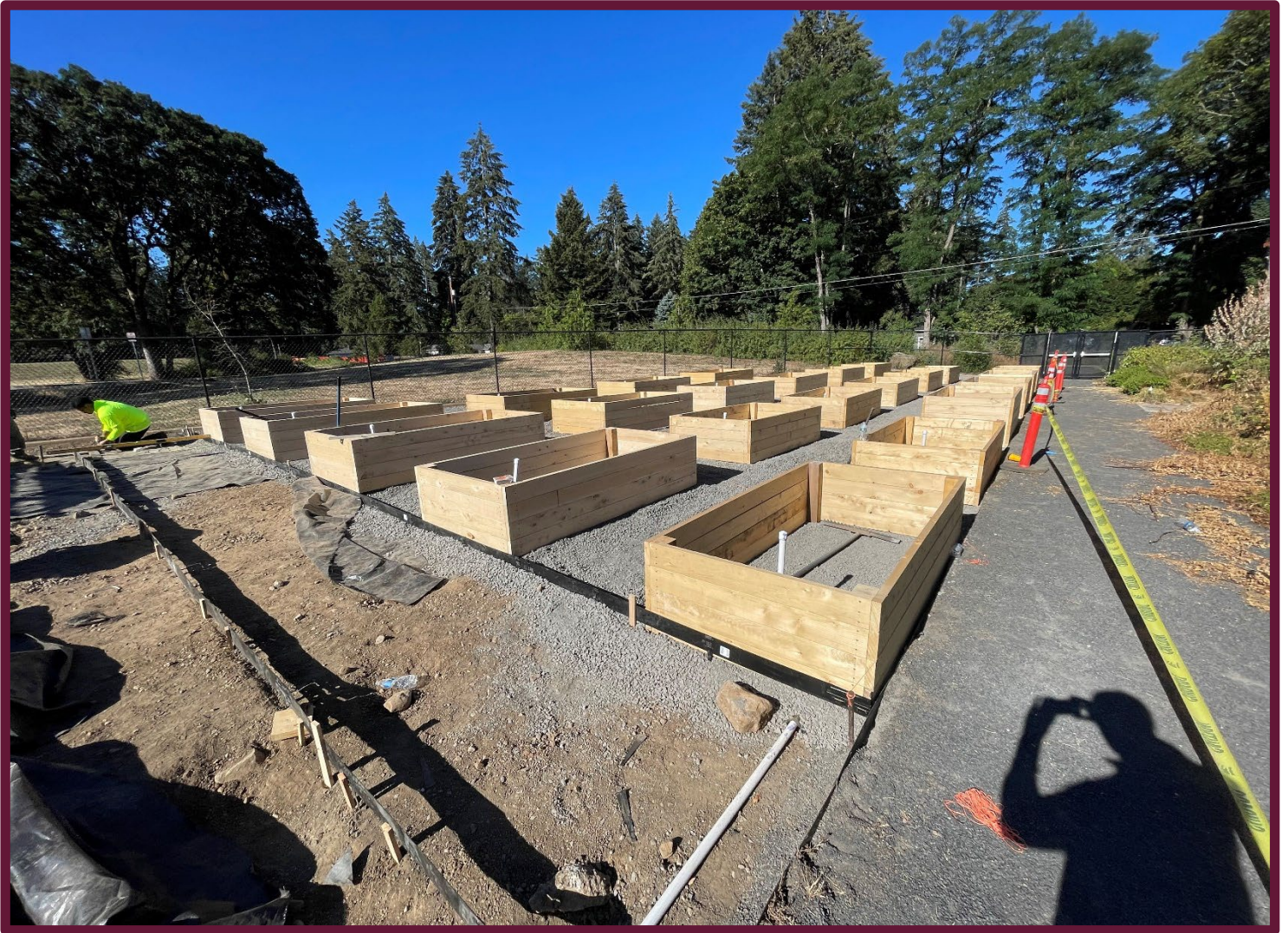
Lakeridge Middle School Garden Planter Boxes
