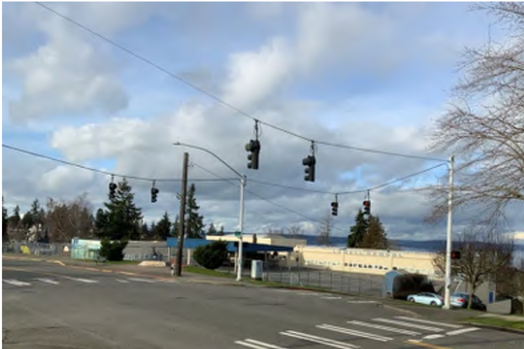
Figure 15: Lowell ES as seen from the corner of 12 th and North "I" Streets. View to the NE.
