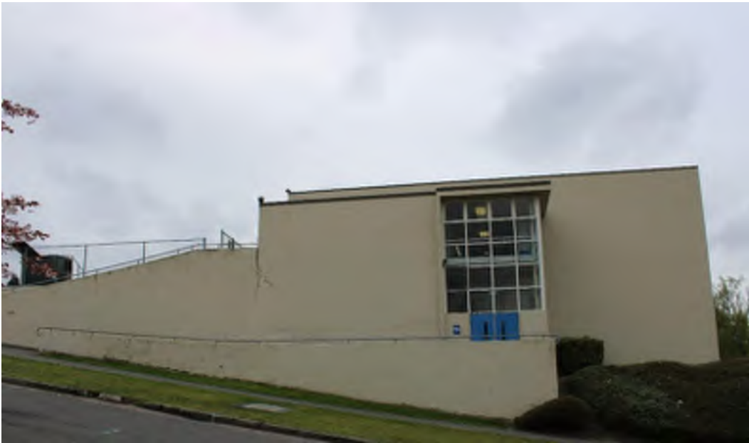
Figure 22: South façade of Lowell ES. View to the N.
