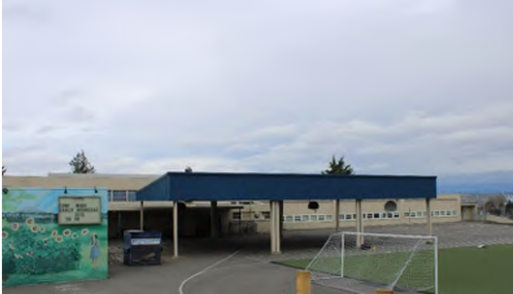
Figure 25: Continuation of west facade. View to the east.
