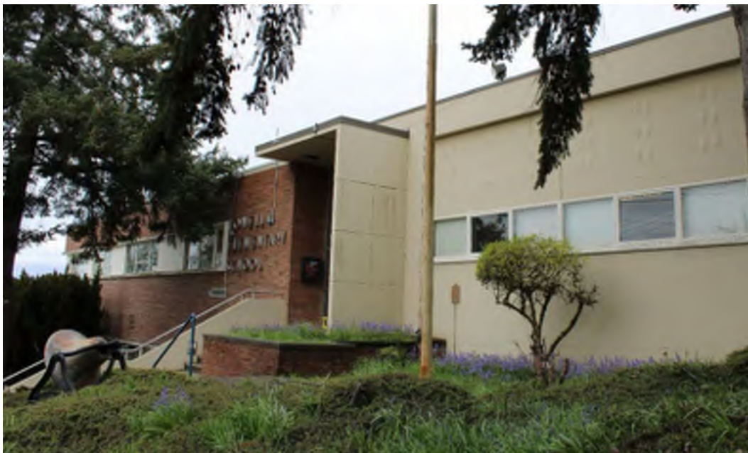
Figure 16: Main entrance to Lowell ES. View to the east.
