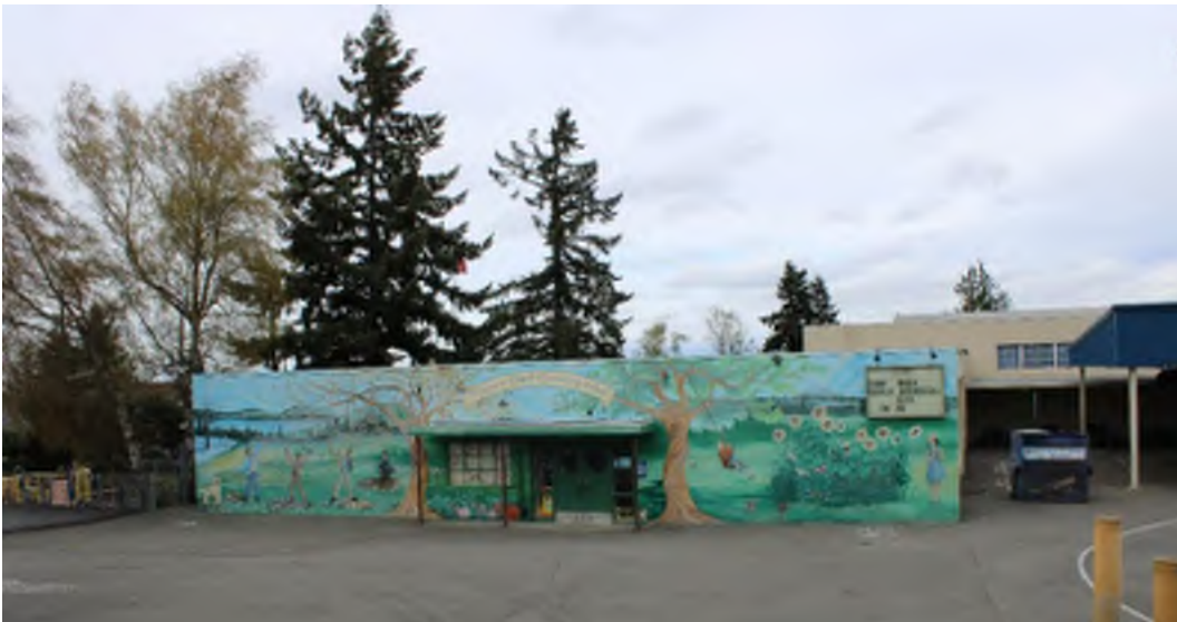
Figure 24: West façade. View to the east.
