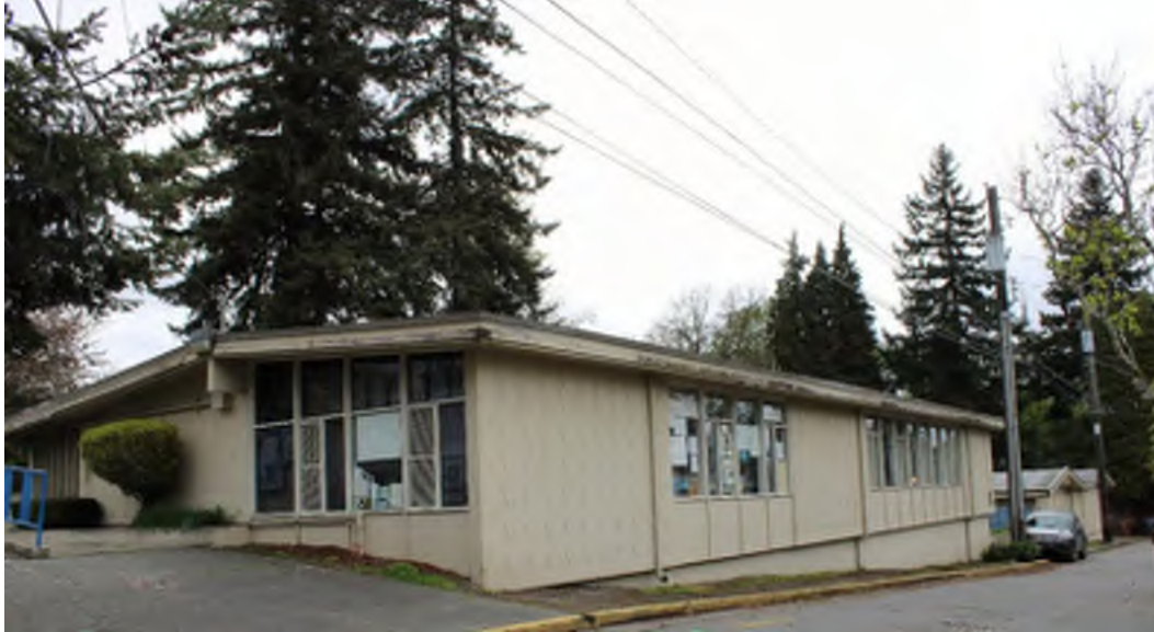
Figure 27: A portion of the quad structures that make up the Lowell ES annex. View to the north.
