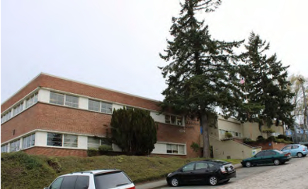
Figure 18: A ¾ profile of primary façade. View to the SW.
