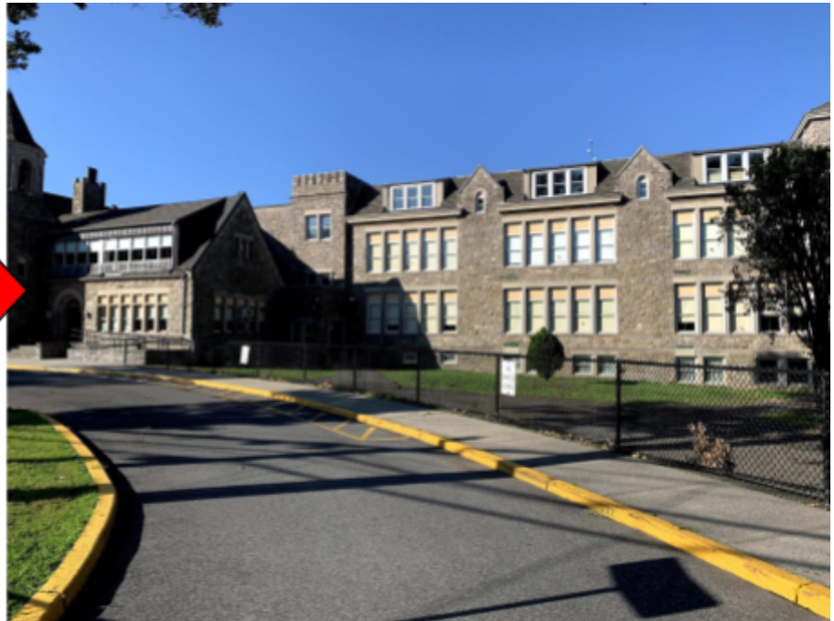
Broadway side of Parsons
