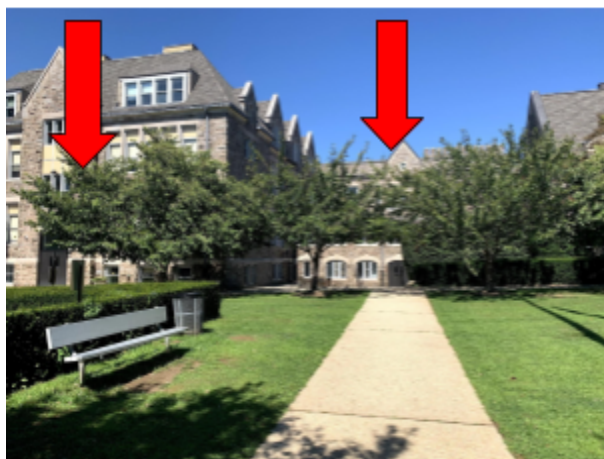
Halstead Avenue side of Parsons
