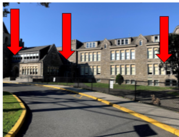
Broadway side of Parsons
