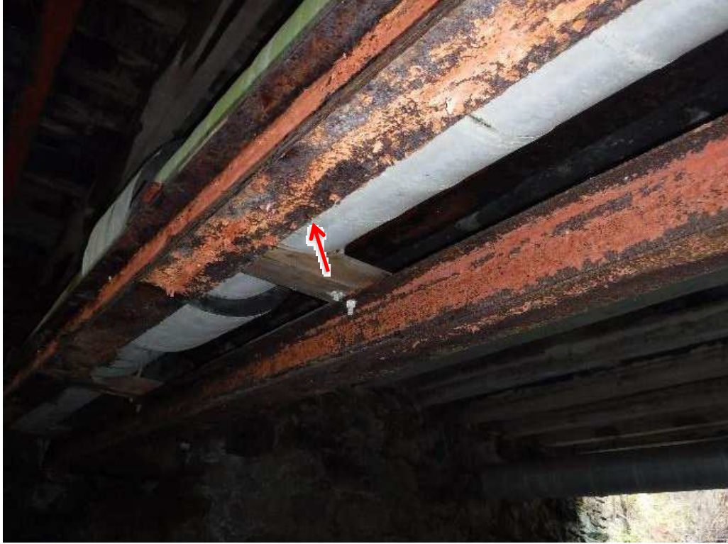
Photo 9: Paint failure, section loss, and bottom flange delamination to the beams supporting Pipe 3
