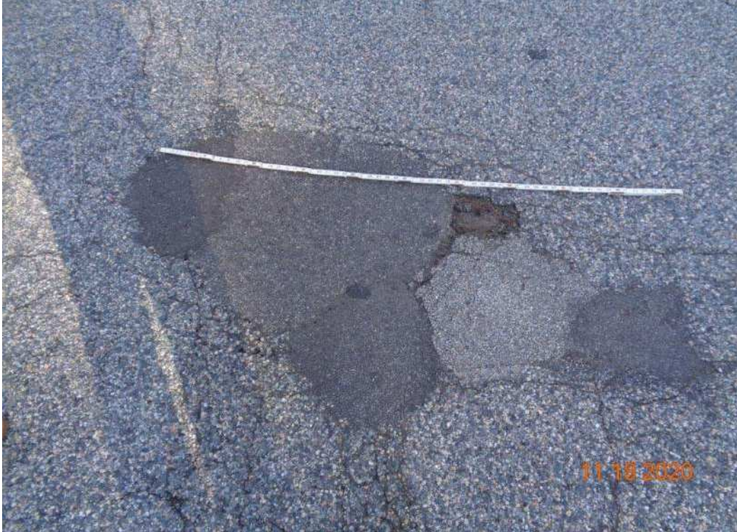
Photo 13: Area of asphalt patching near travel way centerline at Abutment 2, looking north
