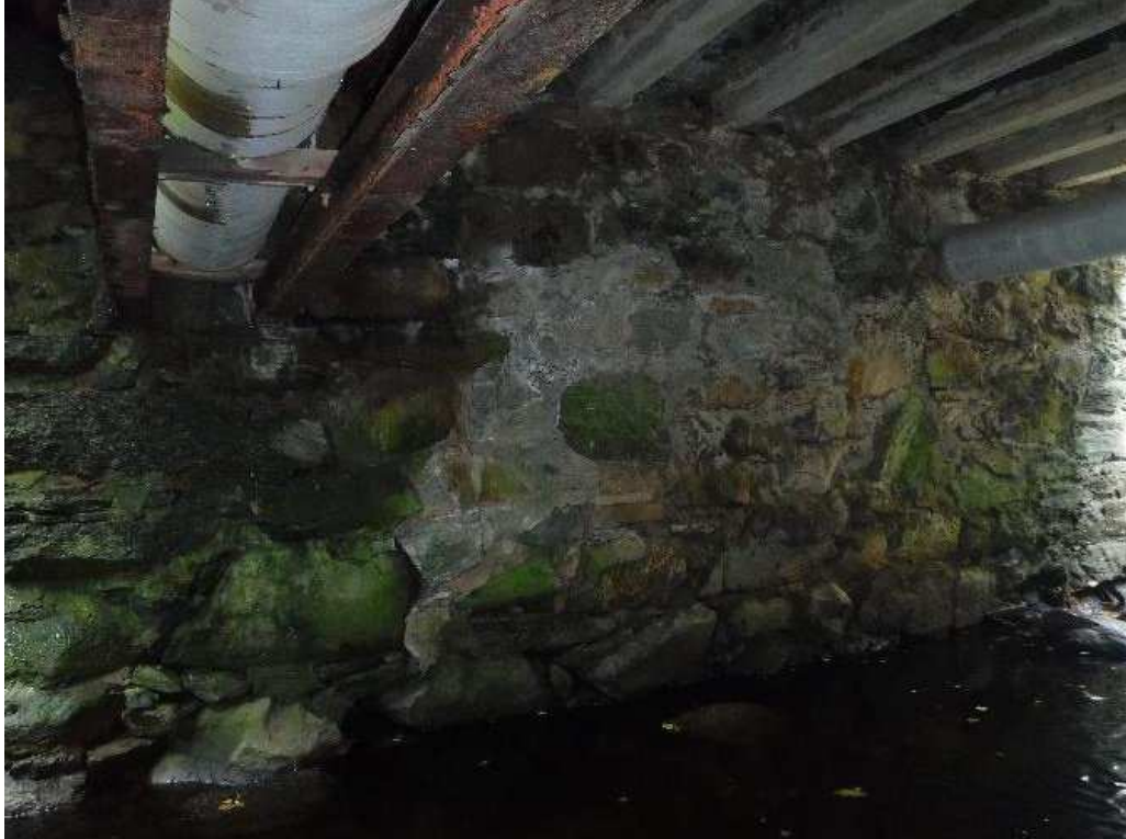
Photo 15: Minor voids and cracks in the north abutment
