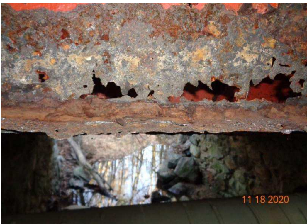
Photo 28: Girder G1 bottom flange near midspan, looking to east
