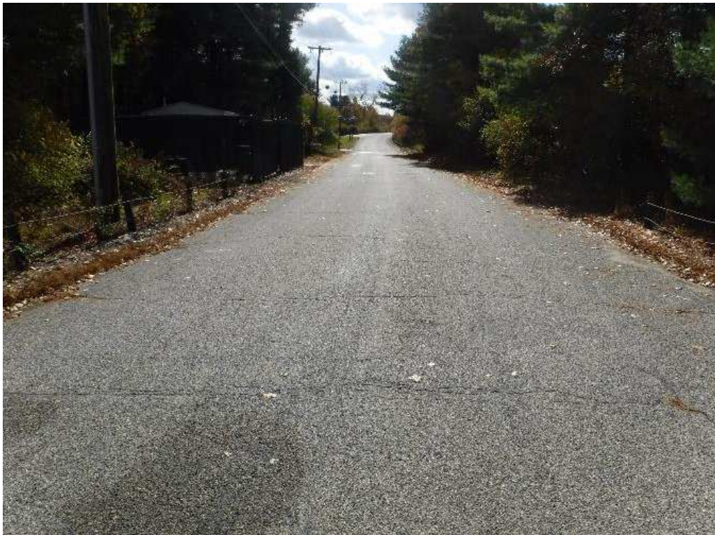
Photo 10: Widespread asphalt cracks, minor settlement, wheel line rutting, and debris accumulation at curbs on the north approach
