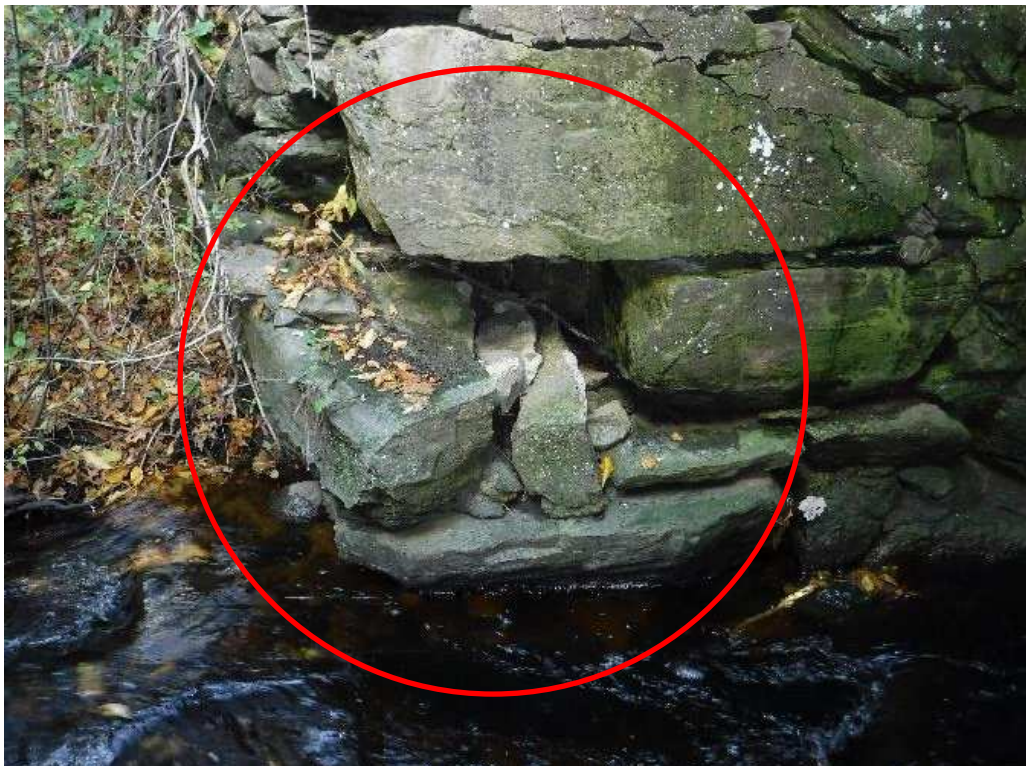
Photo 16: Partial abutment collapse at the northwest abutment corner due to undermining
