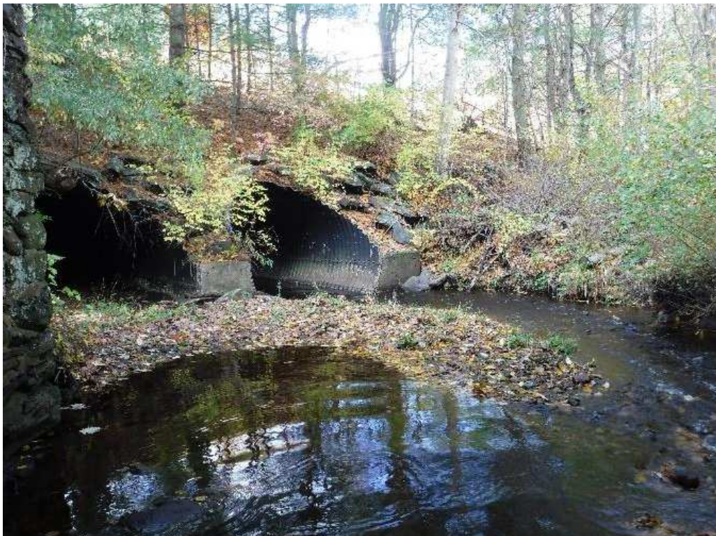
Photo 18: Restricted waterway due to accumulation west of the bridge
