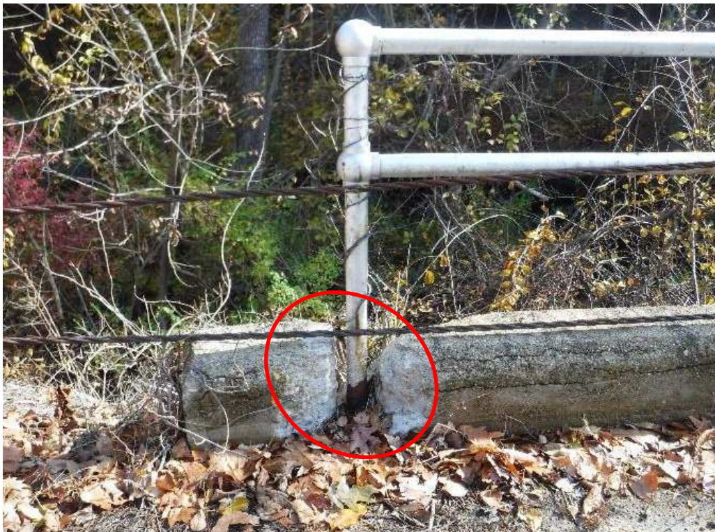
Photo 6: Hole in curb, and rusting and unanchored bridge rail post at the northeast corner
