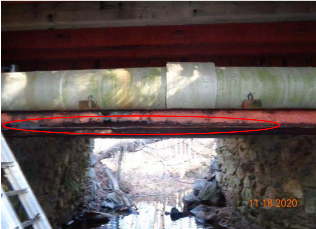
Photo 21: West utility support beam below Girder G3, looking to east
