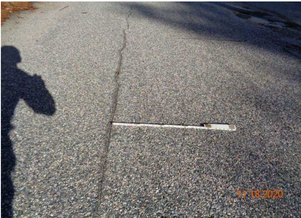
Photo 14: Longitudinal crack in asphalt wearing surface in southbound travel lane, looking to Abutment 2
