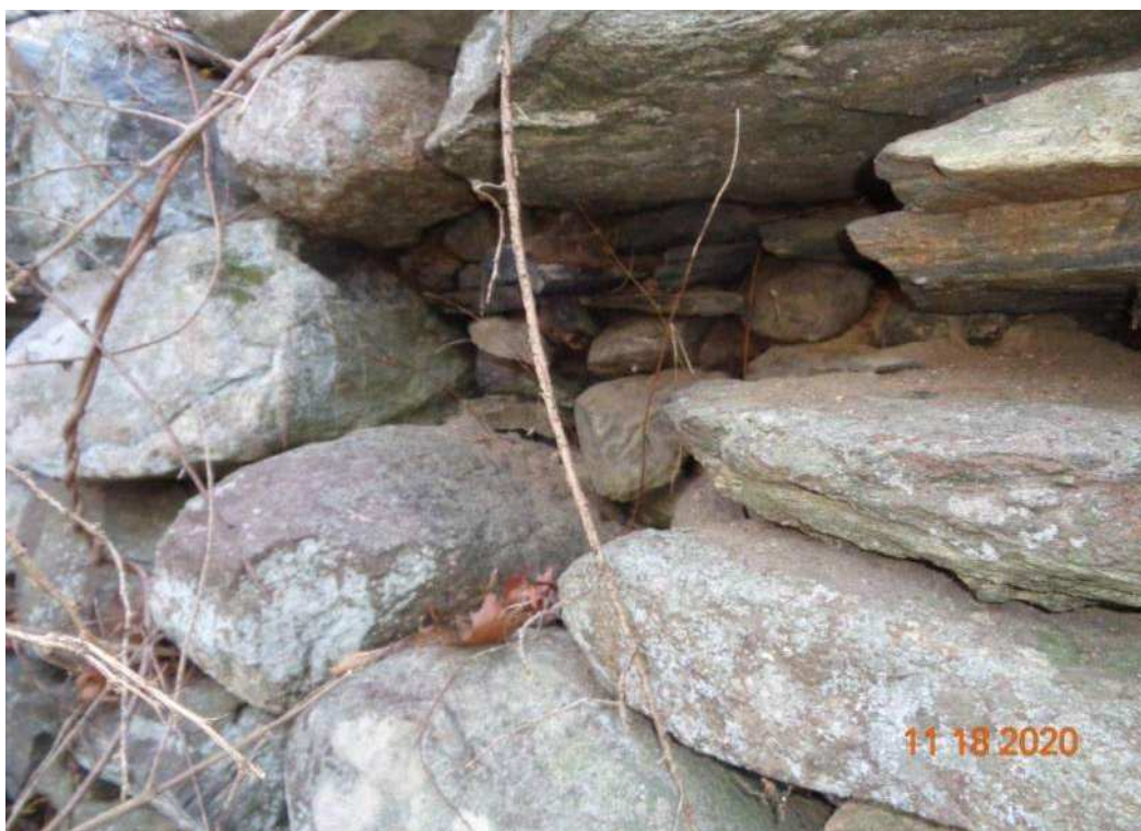
Photo 41: Void in Southeast Wingwall, looking south
