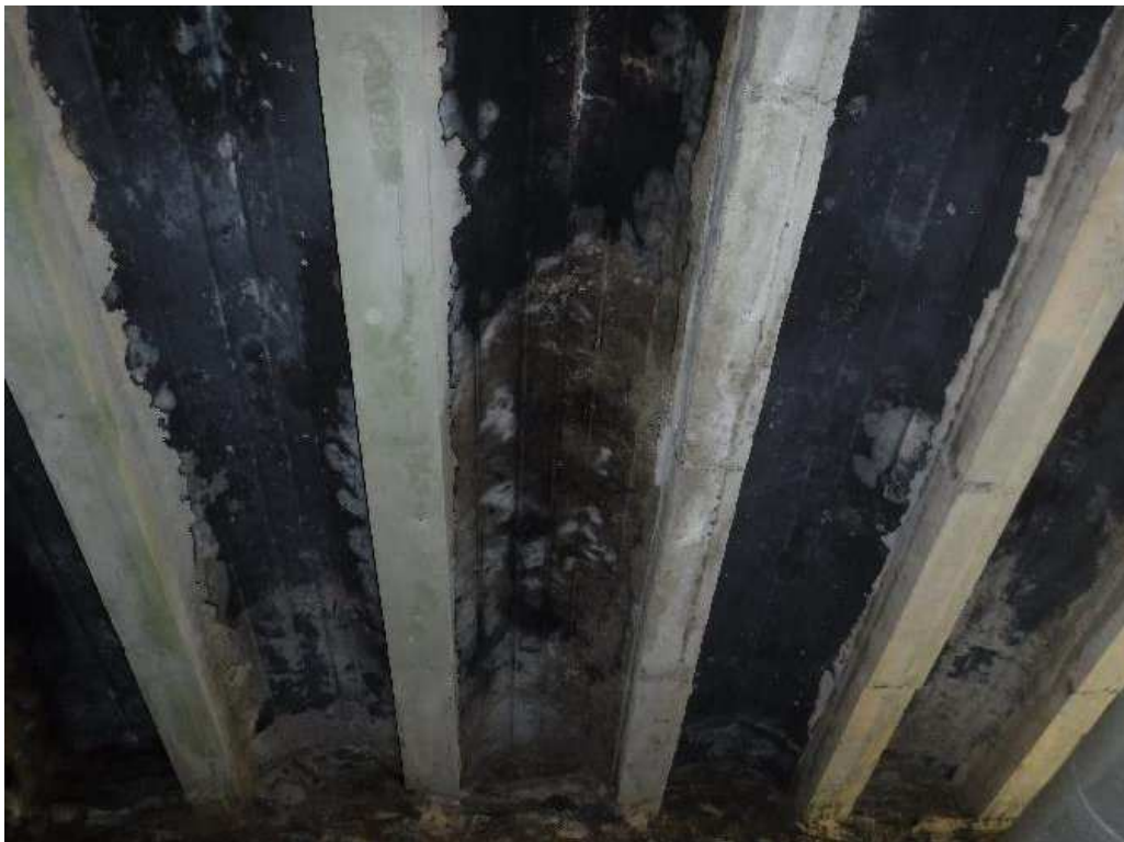
Photo 4: Typical jack arch concrete deck and encased steel beam condition
