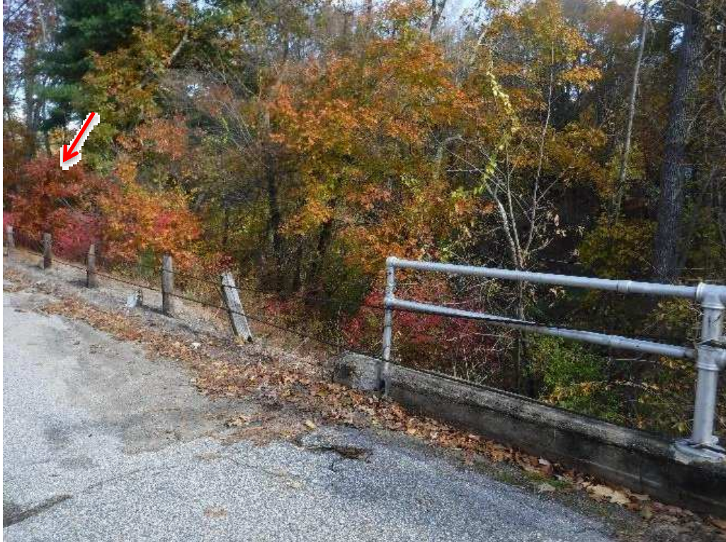
Photo 11: Loose cables and broken posts at the northeast approach railing
