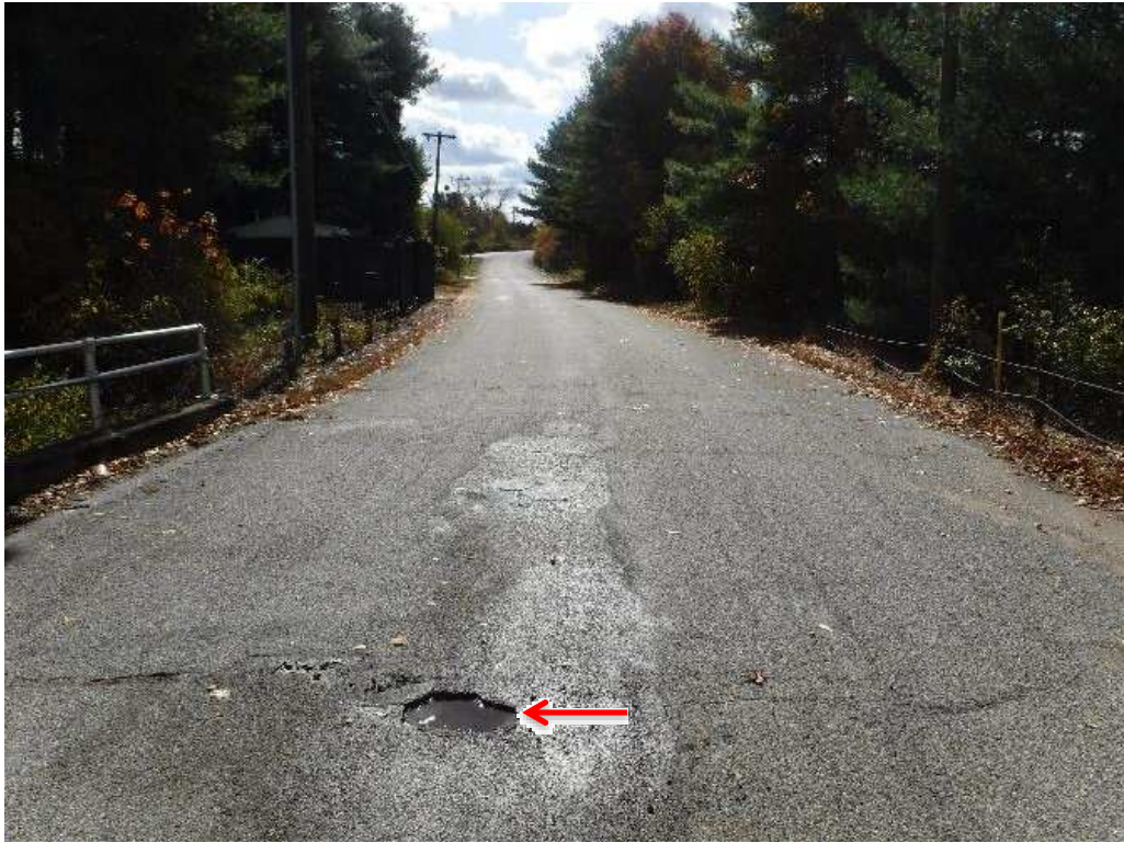
Photo 1: Moderate potholes, patches, and cracks on the bridge wearing surface
