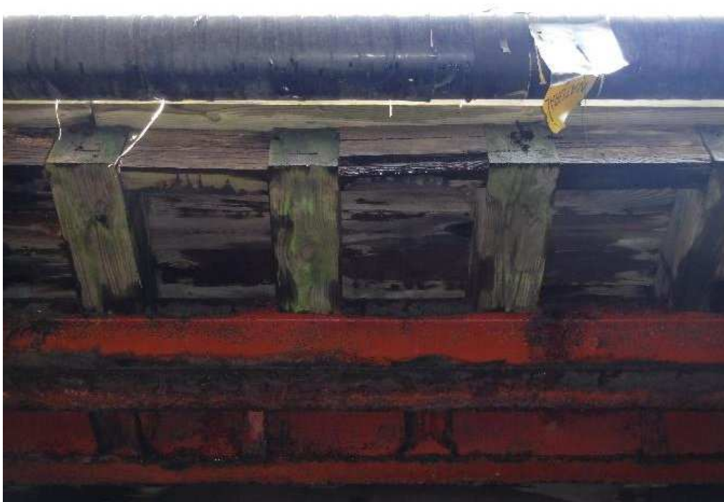
Photo 3: Rotting wood and active leakage on the west fascia
