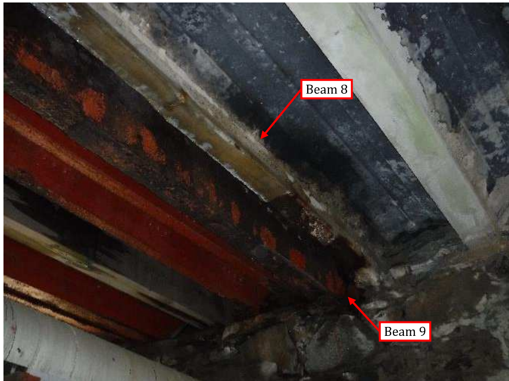
Photo 13: Severe deterioration to Beams 8 and 9
