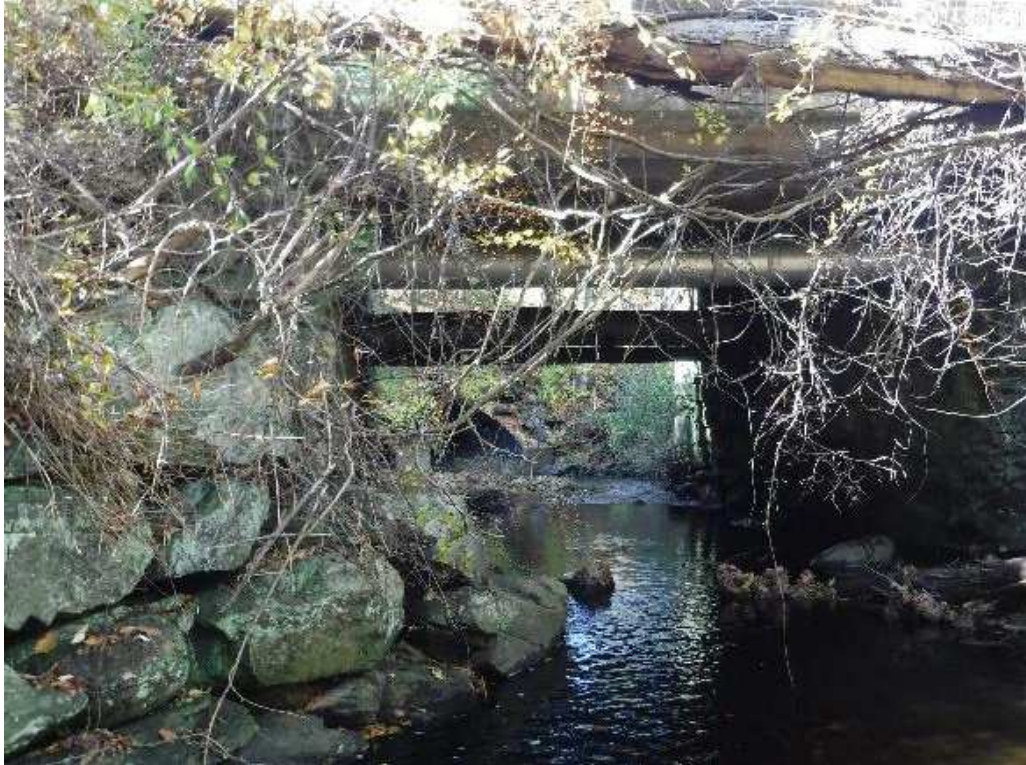
Photo 17: Overgrowth and voids at the northwest wingwall
