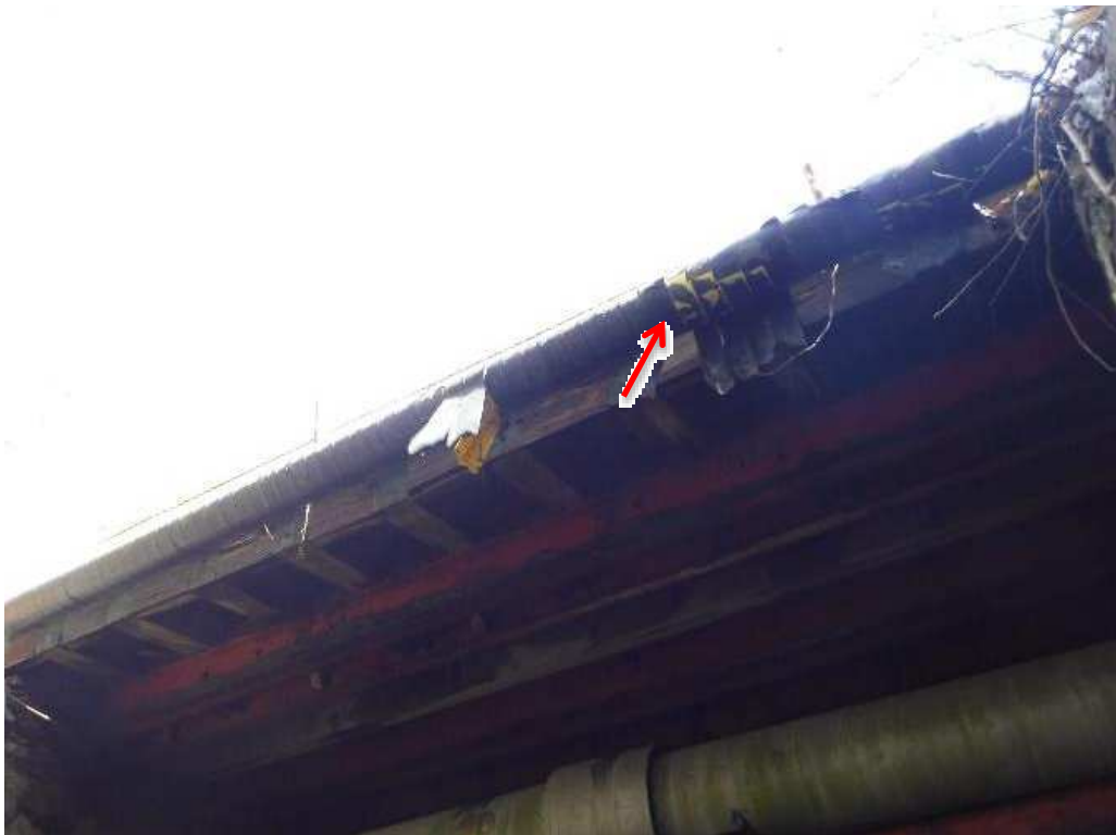
Photo 8: Protective wrapping peeling off Pipe 4
