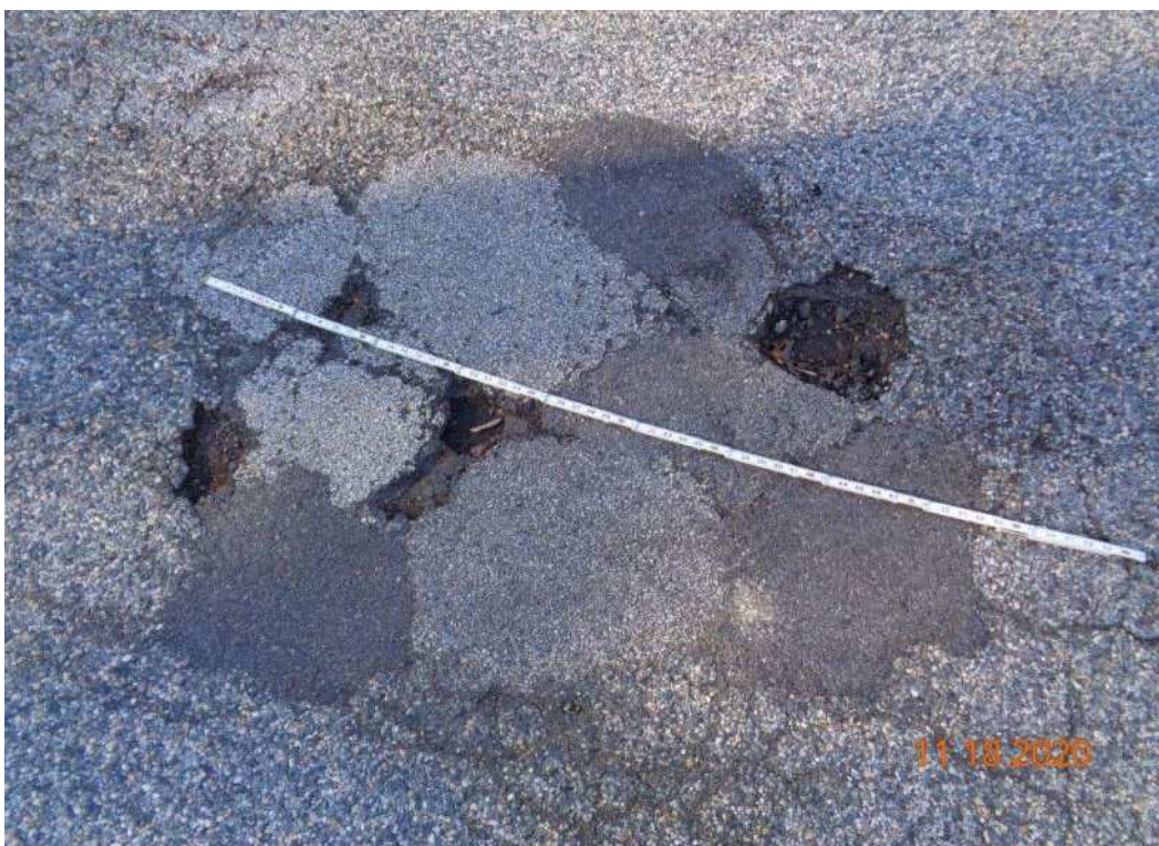
Photo 12: Area of asphalt patching and pothole near travelway centerline, 6 ft. from Abutment 1, looking west
