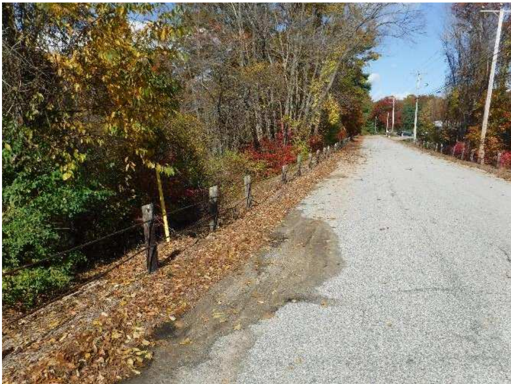
Photo 2: Settlement and debris accumulation at the northwest shoulder
