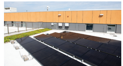
The rooftop garden and solar panels both allow students to go outside and explore how things are grown and how energy is collected and repurposed.
