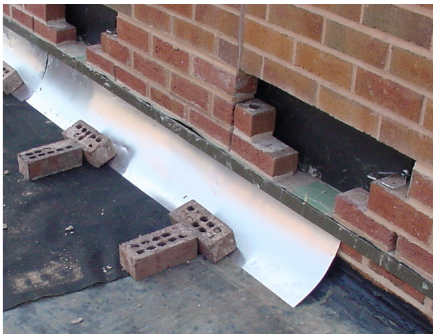
Photo 3 Flashing Installed in Alternating Sections
