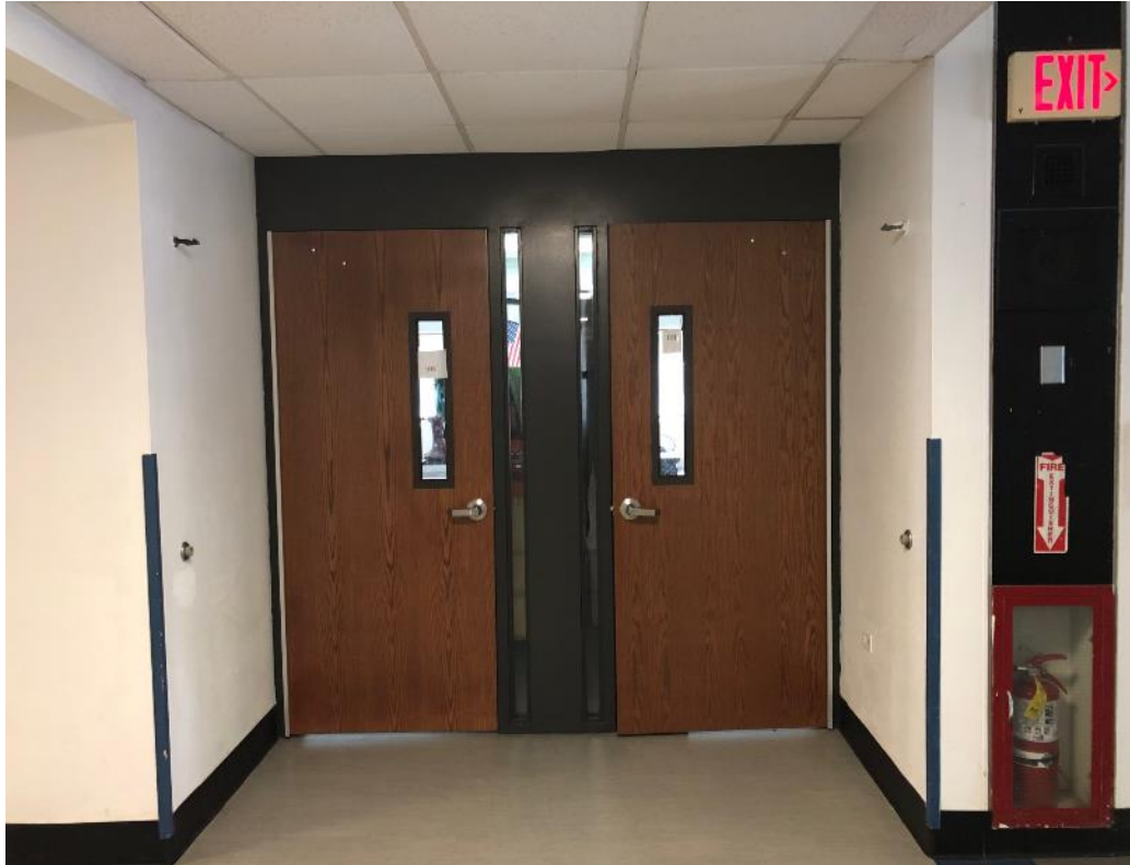
New Doors & Hardware
