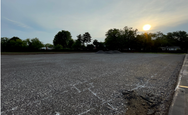
SDS - Subbase Preparation for New Tennis / Activity Courts
