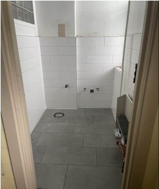
WBS - Classroom Bathroom Floor & Wall Tile Install
