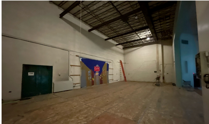
SDS - Auditorium Stage Flooring Protection + Stage Rigging / Lighting Removed
