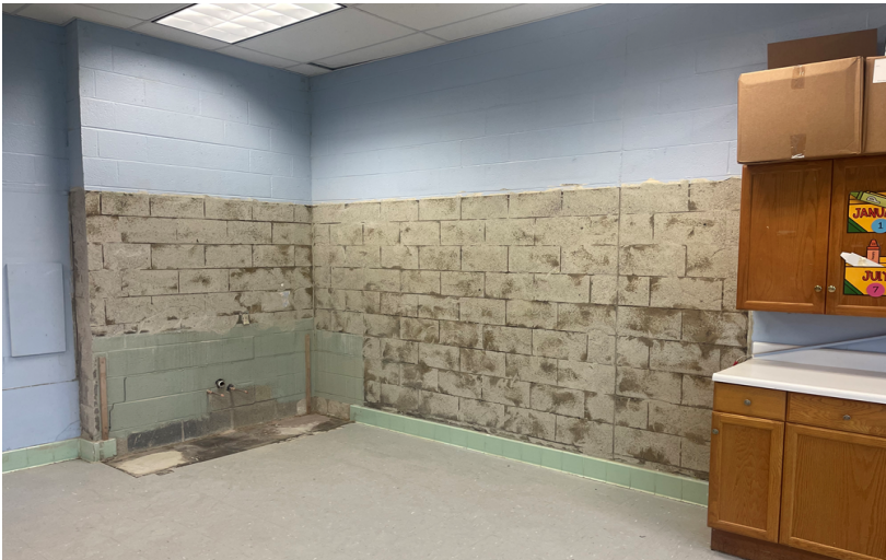
WBS - Classroom Casework Replacements - Demolition Complete
