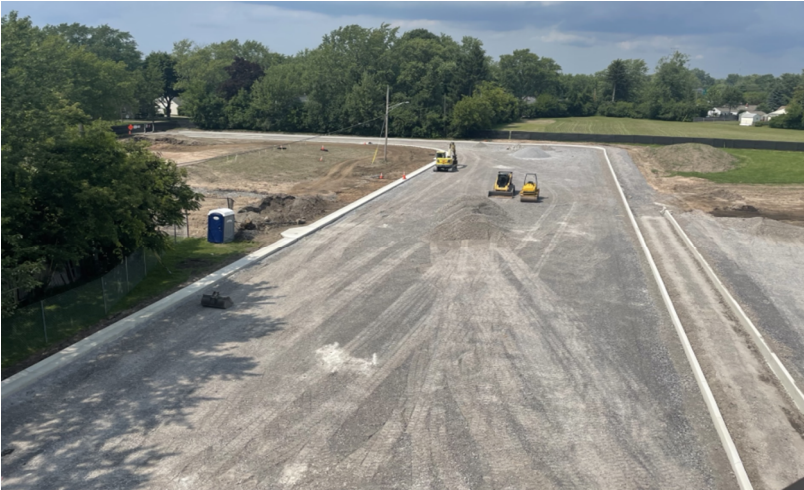
SDS - New Bus Loop - Stone subbase with concrete curbs and gutter
