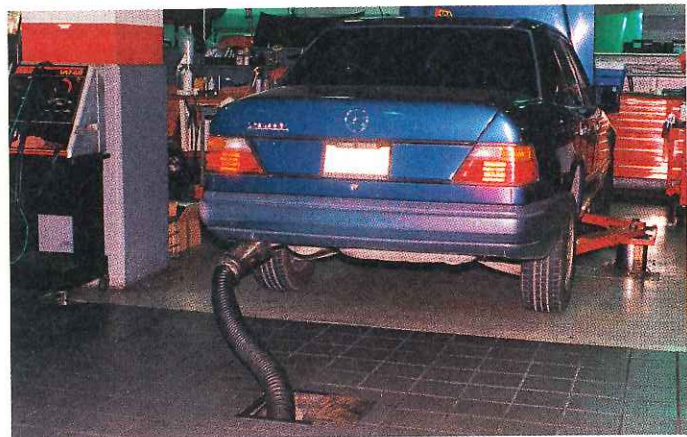
Figure 3.17 Use an exhaust ventilation system when working around a running engine. (Courtesy of Tim Gillies)
