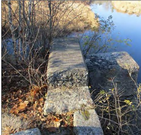
Station No. ~100+00_West abutment of former Nonesuch River railroad bridge and tie-in location to existing trail – looking Northwest
