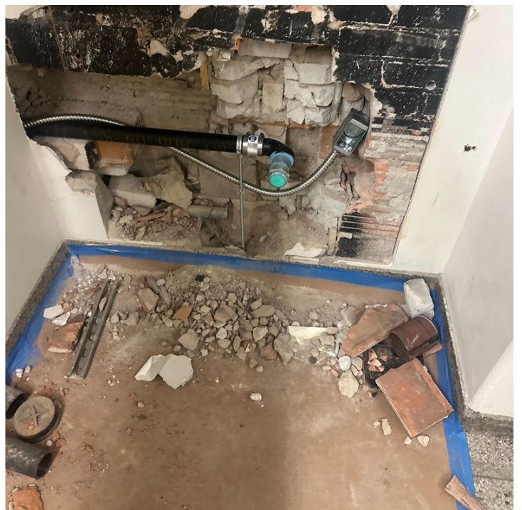
From top left: New waste pipe behind concrete wall; new water supply piping; connecting existing sinks to new piping; drinking fountain piping (July 2024)
