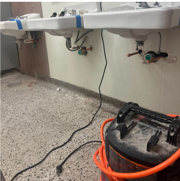
From top left: New waste pipe behind concrete wall; new water supply piping; connecting existing sinks to new piping; drinking fountain piping (July 2024)
