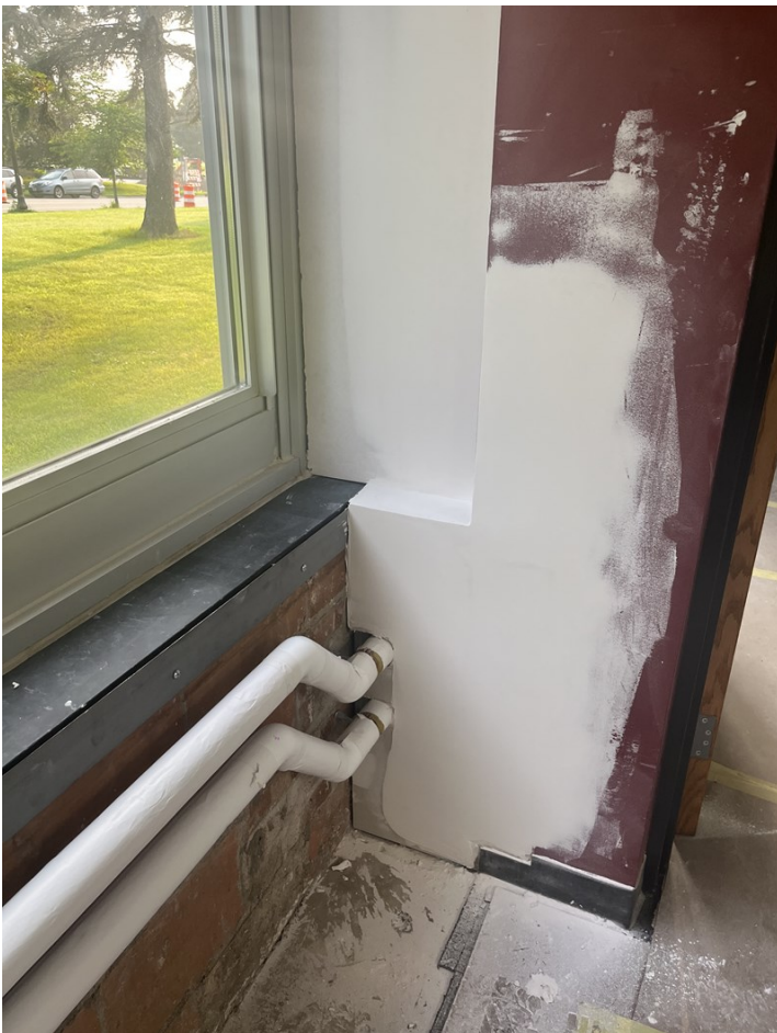
From top left: Ductwork in corridor; ceiling grid and break metal; drywall patching for hydronic risers; finned tubed radiation with covers (July 2024)
