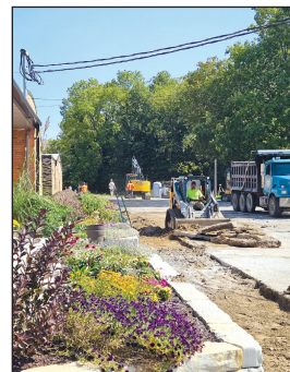
CONCRETE WORK AT THE ELEMENTARY SCHOOL
