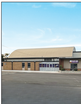
NEW ROOFING INSTALLED OVER THE ELEMENTARY GYM
