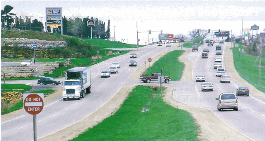
To make a left turn from a side road onto a multilane highway, a median strip provides a safe place to wait for a gap.
