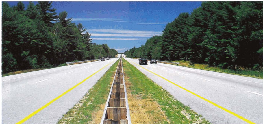
A median strip safely separates high-speed traffic that moves in opposite directions.
