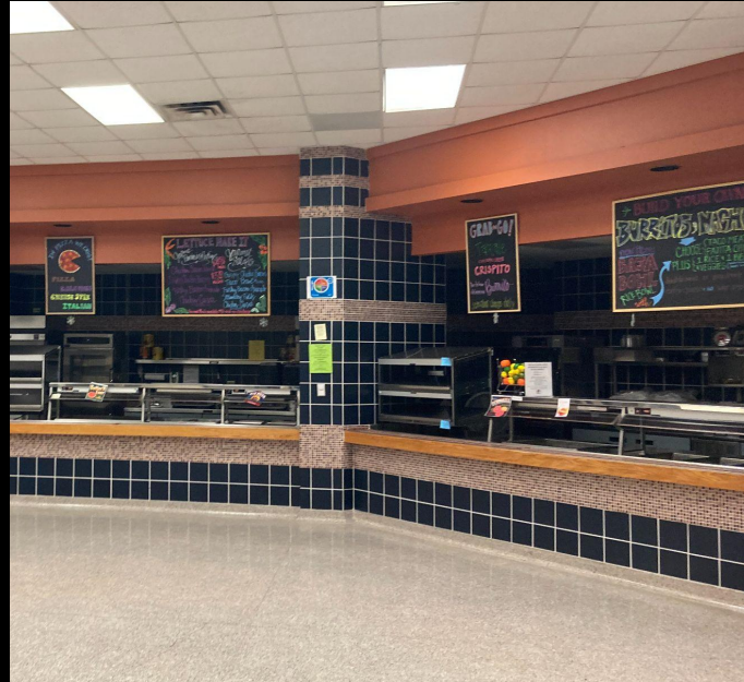
KITCHEN SERVING AREA: New wall tile, counter tile, paint on bulkhead
