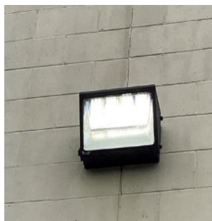
Wall-mounted LED fixture
