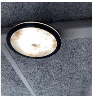
Under canopy LED fixture
