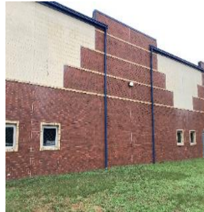
Exterior wall with brick facade
