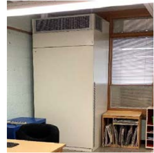
Single packaged vertical unit for classrooms
