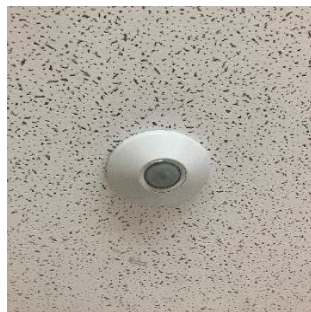
Ceiling-mounted occupancy sensor
