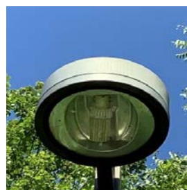
Pole-mounted fixture with LED corn shaped lamp
