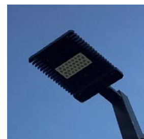
Pole-mounted LED fixture
