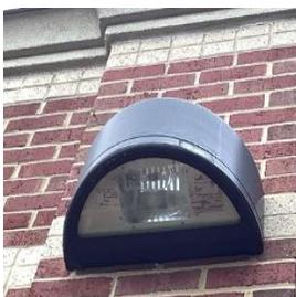
*Wall-mounted fixture with metal halide lamp*
