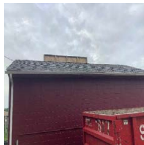
Walls and roof
