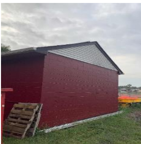
Walls and roof
